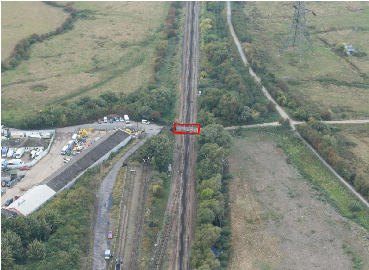
Figure 3 - Aerial photograph of Cattle Creep Under Bridge looking west (October 2016).
