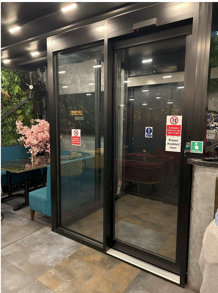
Figure 12- Acoustic lobby into the enclosed courtyard area. Operates on a push button and automatic sensor. Lobby is fully enclosed including the ceiling.
