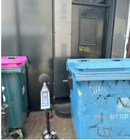
Figure 4- Fire exit pointing towards R1 on Manor Road.
