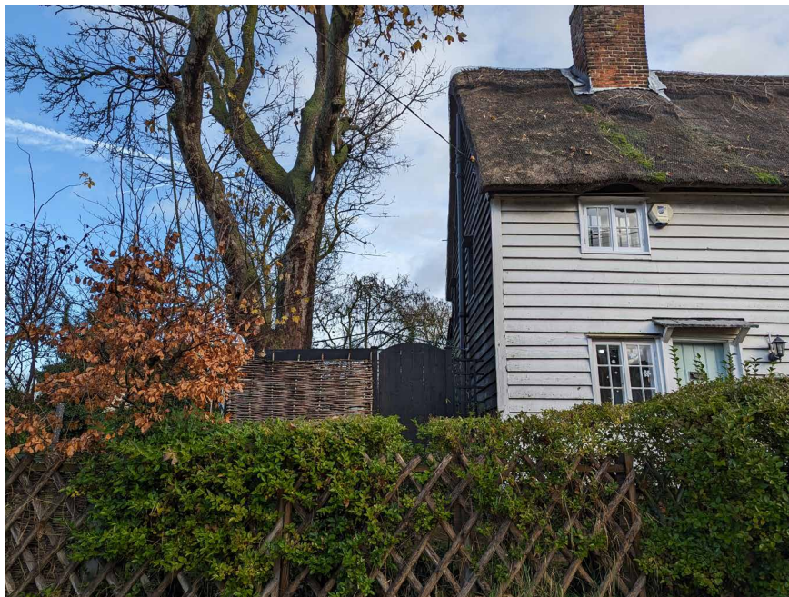
View from Church Street
