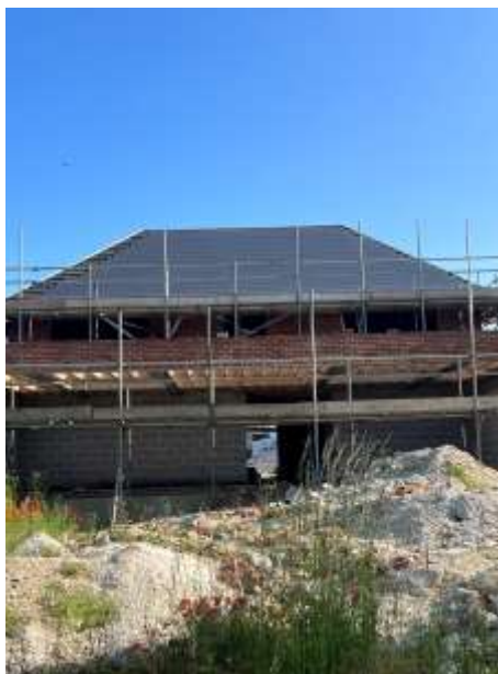
REAR VIEW OF PARTIALLY COMPLETED NEW DWELLING
