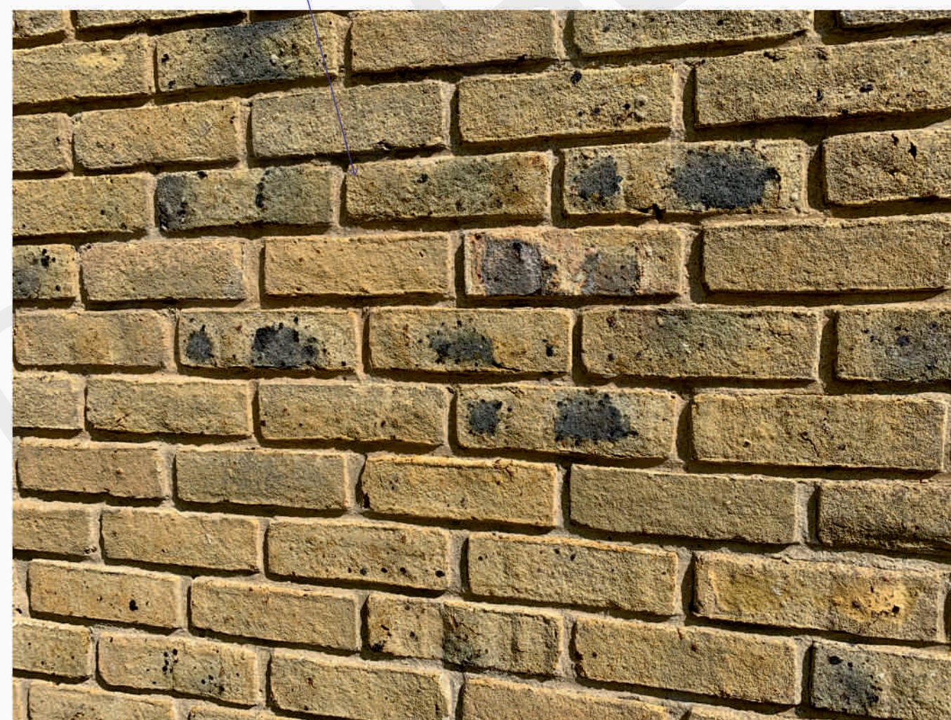
PHOTOGRAPH CLOSE UP OF EXISTING FACING BRICK MATCHING PROPOSED BRICKWORK FOR THE STABLES
