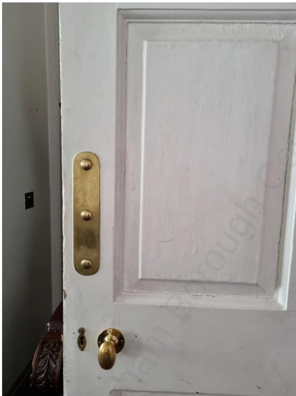
Photo 22: Representative detail image of existing door fixtures, second door to Old Court Room
