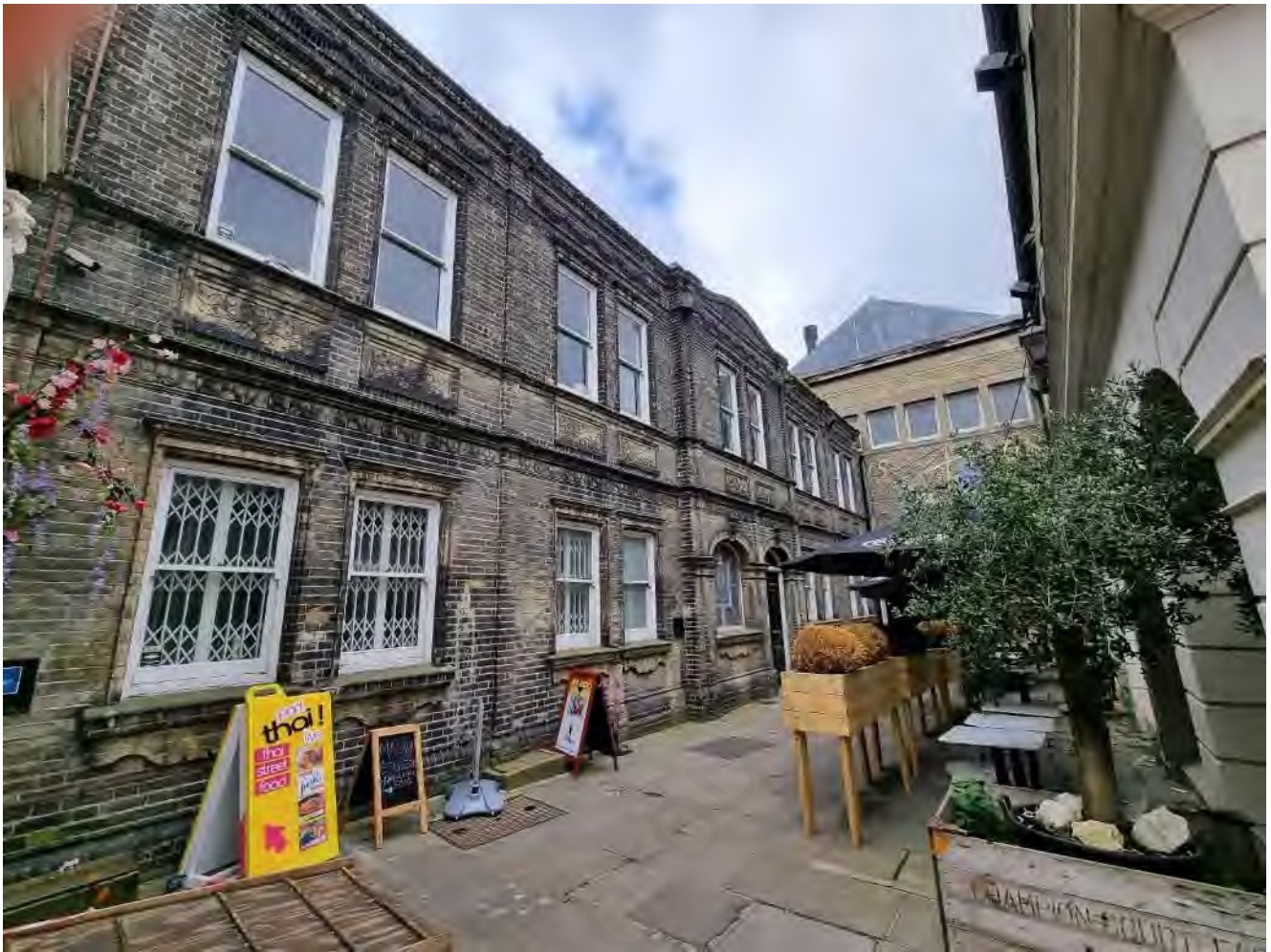
Photo 6: Southern wing facing south west
