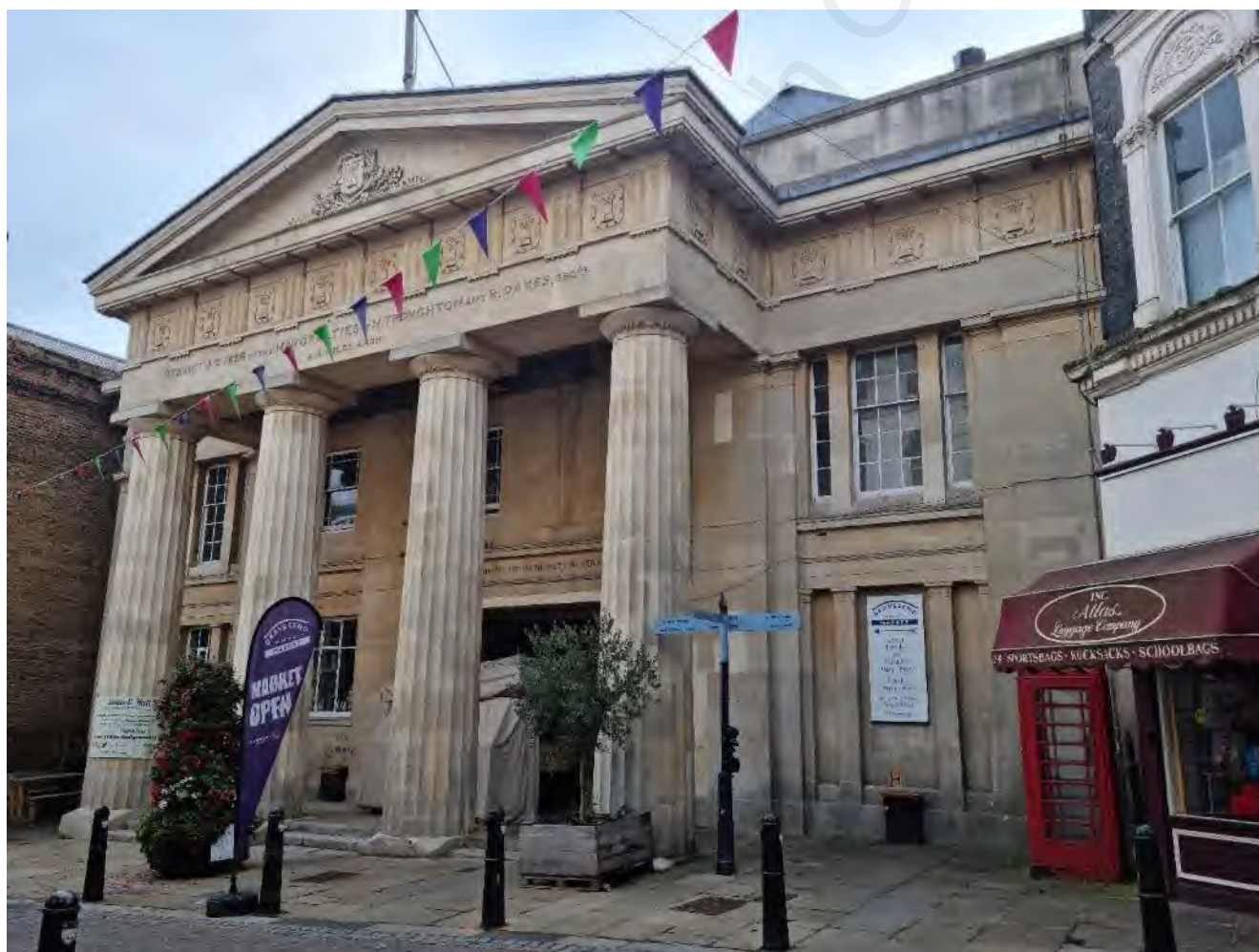
Figure 2: General view of Gravesend Old Town Hall facing north east from High Street
