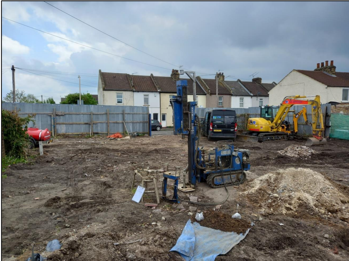
Drilling Rig and soils encountered in BH01
