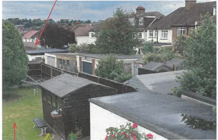
Views from the back of 1 Dennis Road showing flat roofed garages
