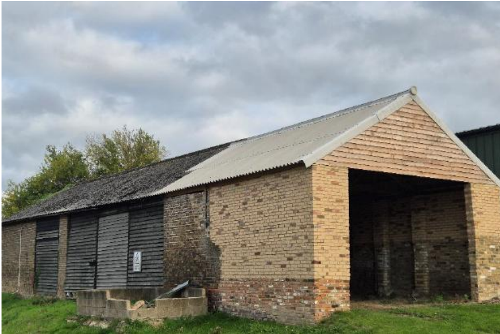
Figure 1 – photograph of existing building (DSA).
