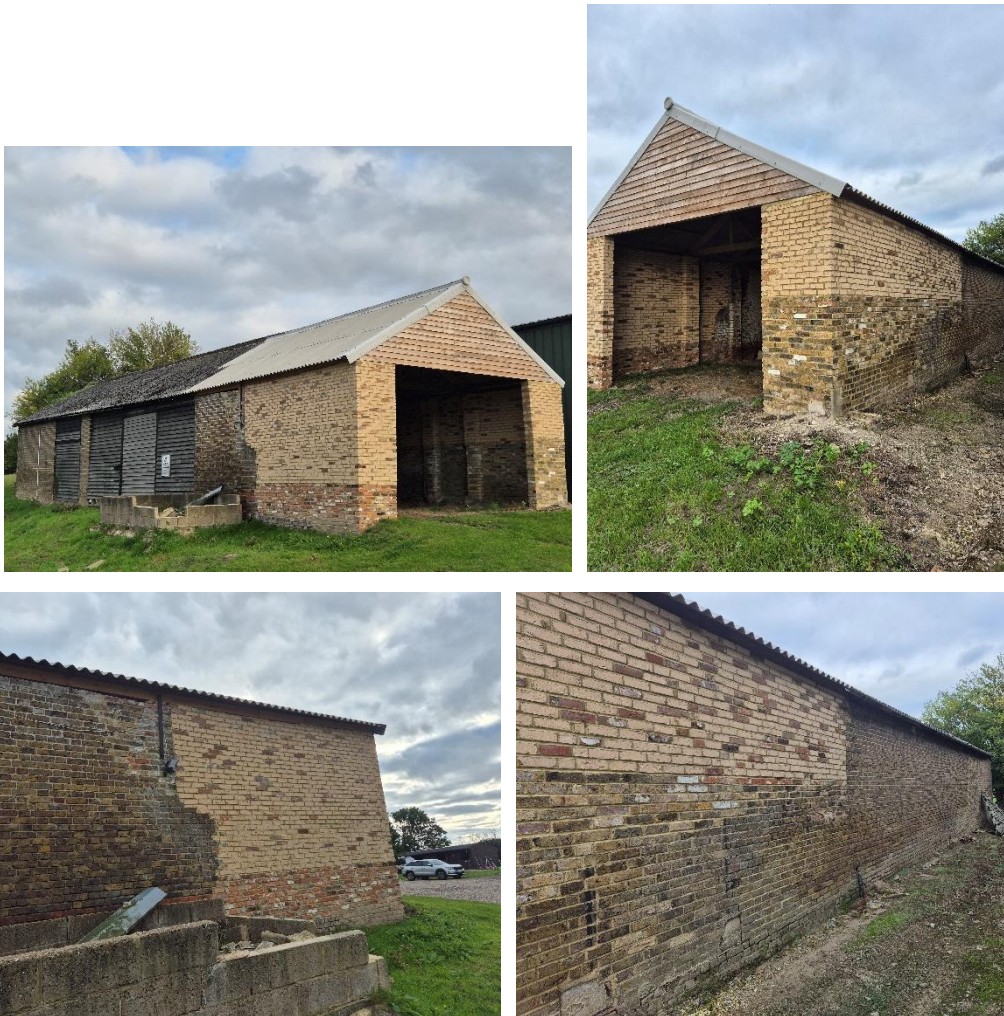
Figure 1: Photographs showing the rebuilt section of the barn
