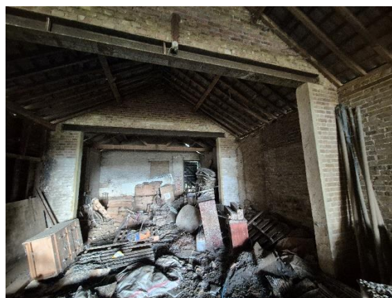
Figure 6: Beam in situ supporting gable brickwork between bays
