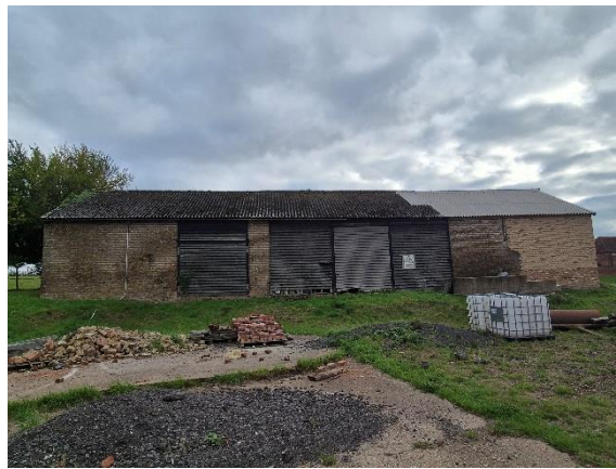
Figure 7: Photographs of the Barn exterior (West elevation, South Elevation, East elevation, North elevation)
