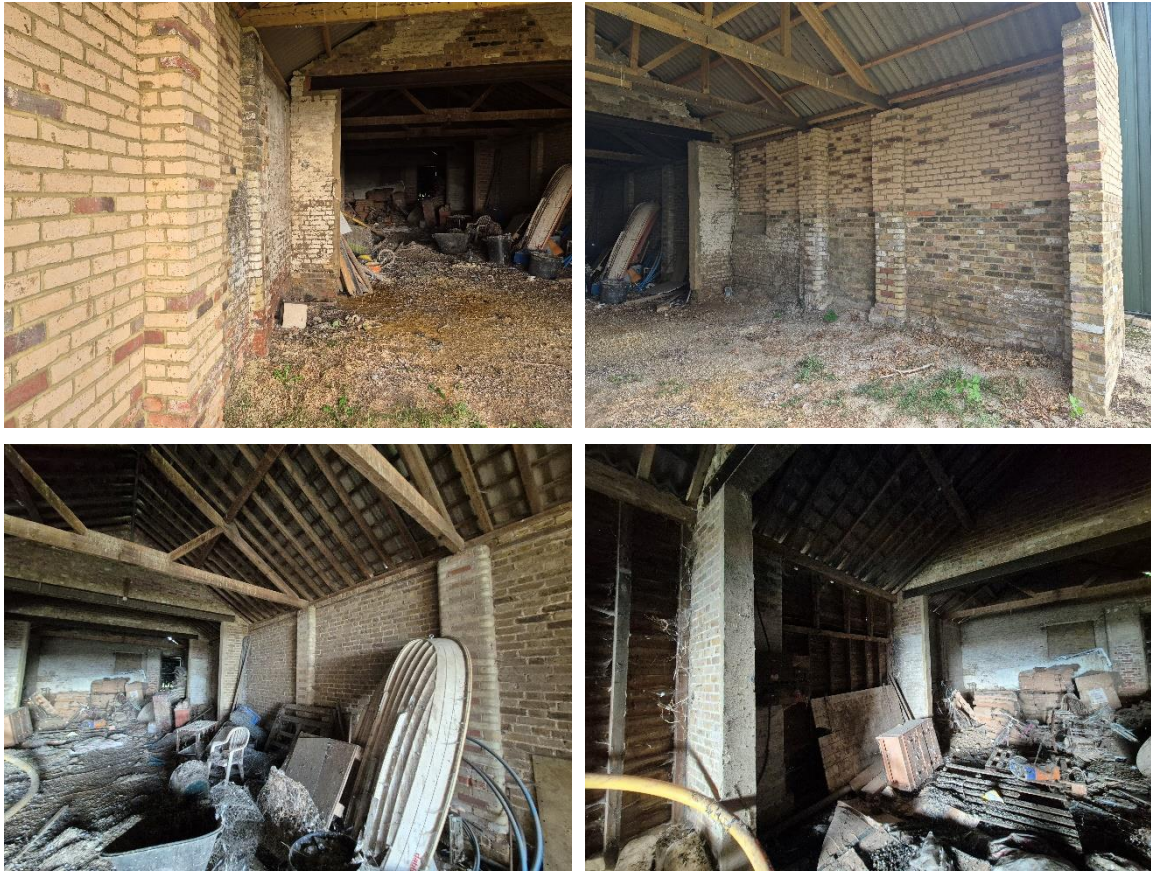
Figure 2: Photographs showing the buttresses and pier walls within the barn
