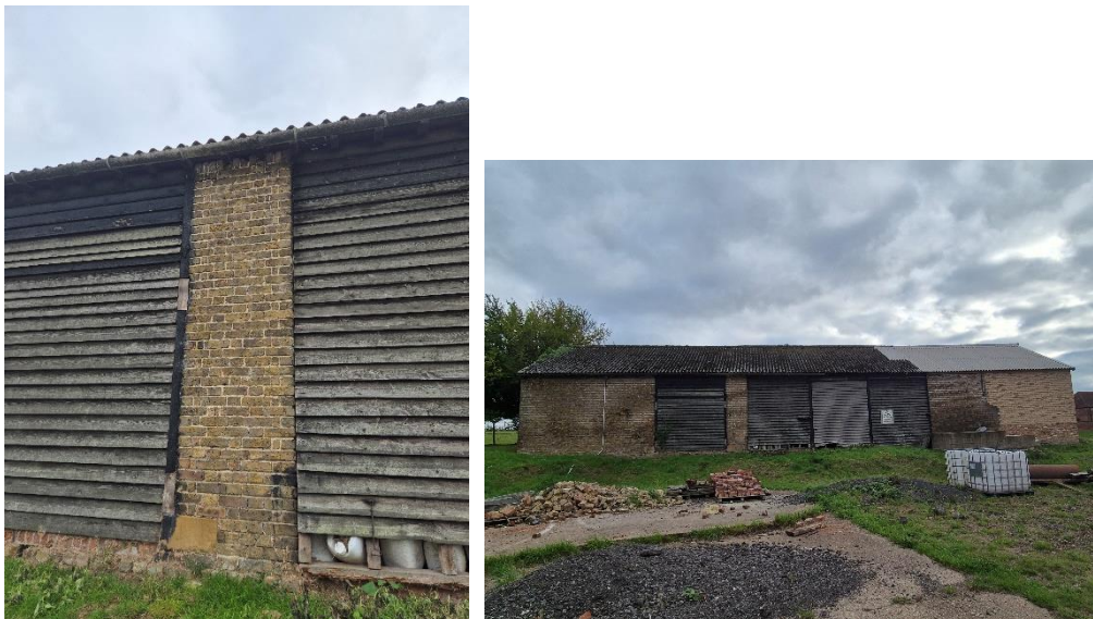
Figure 3: Timber infill panels in the North Elevation
