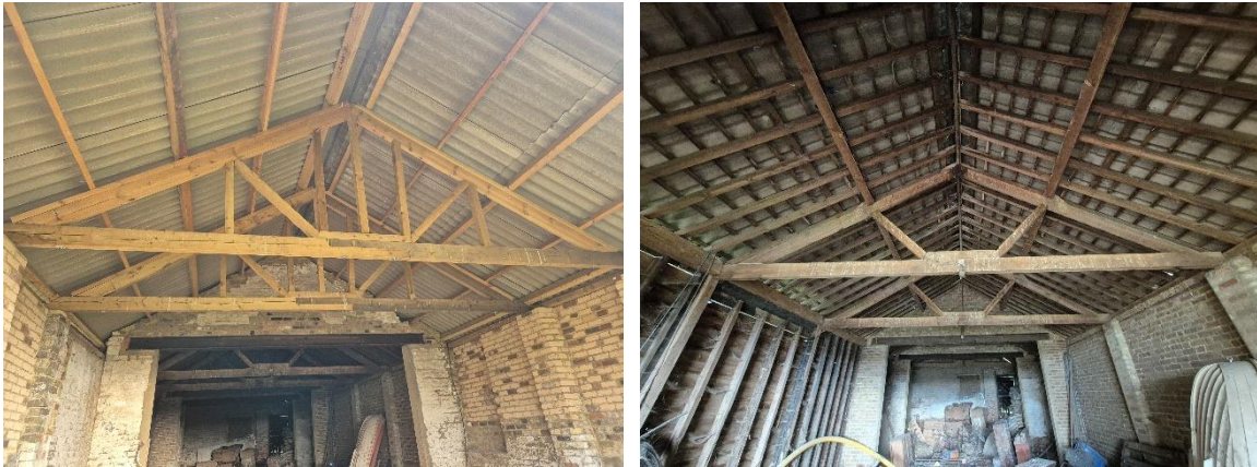
Figure 5: Modern trusses (left) original trusses (right)
