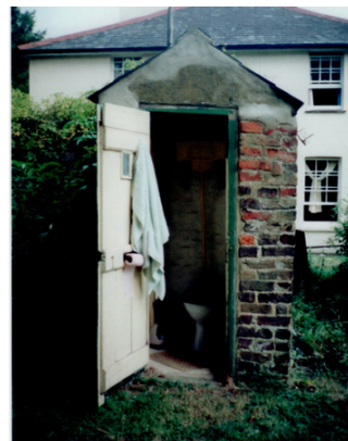
Demolished toilet block
