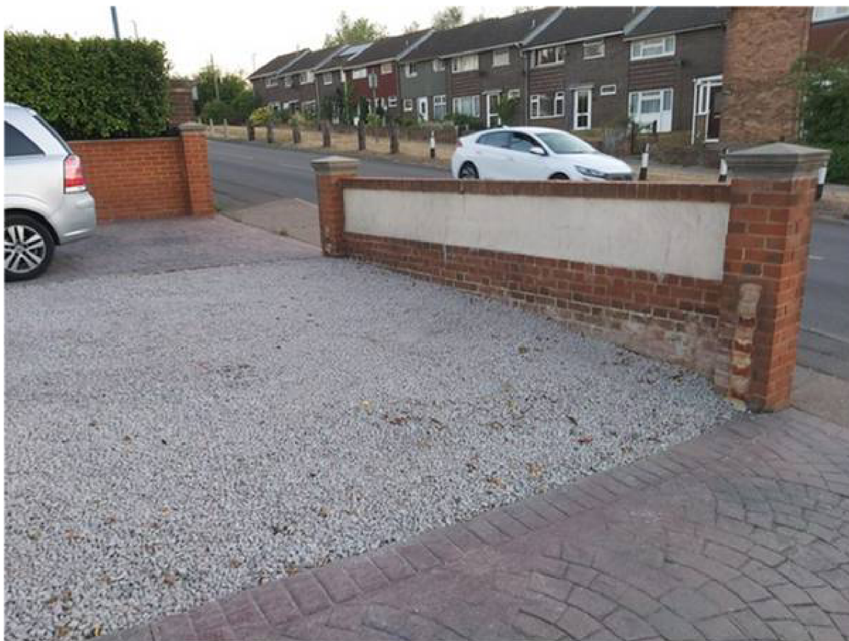
Figure 1: Front boundary wall as built in 2003.
