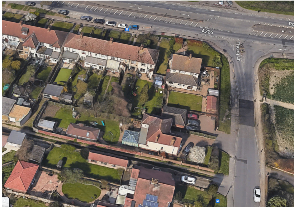
Fig 007 Aerial view of site looking North
