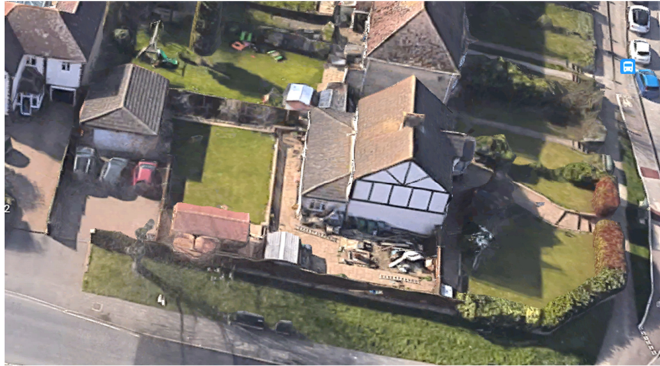
Fig 009 Aerial view of site looking west
