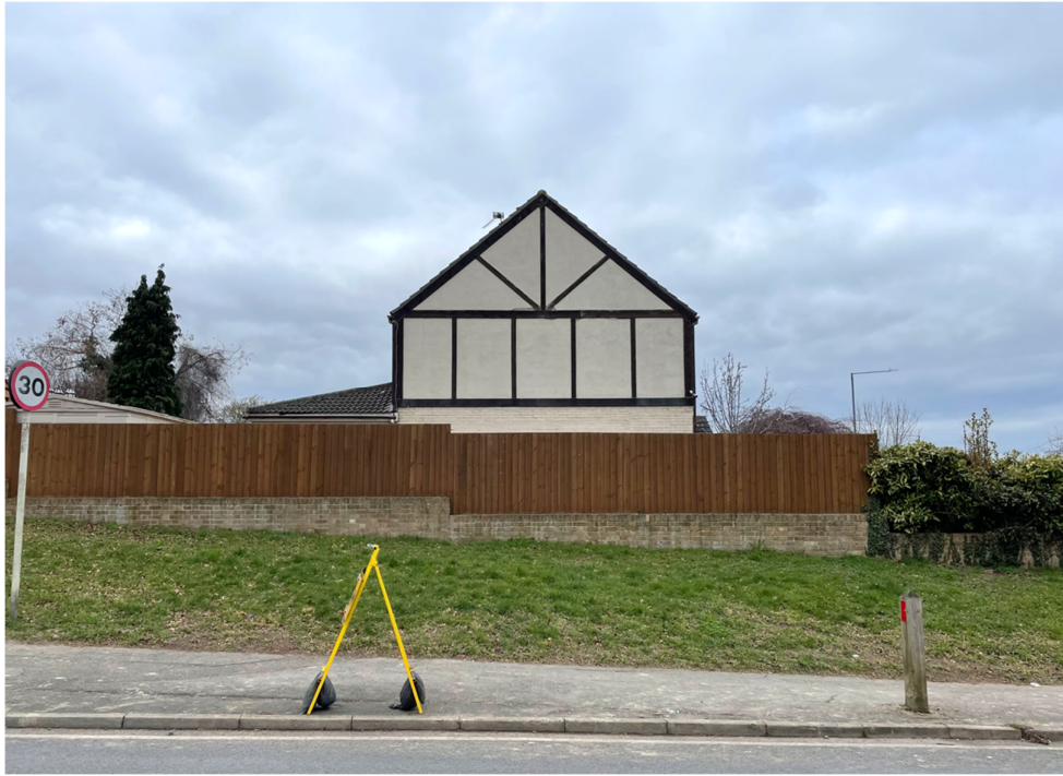
Fig 005 Poor presentation of existing east elevation
