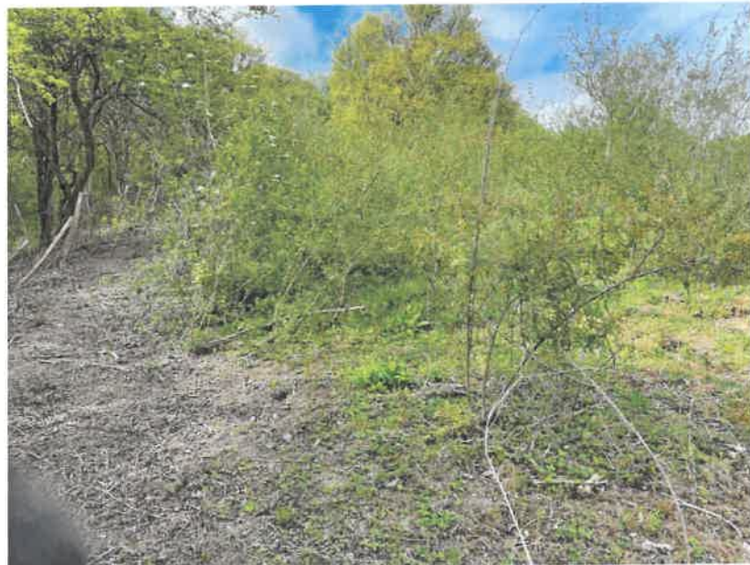
PARTIAL CLEARANCE OF INVASIVE SCRUB TO ENABLE ACCESS FOR REPLACEMENT OF FENCE POSTS (8/5/23)
