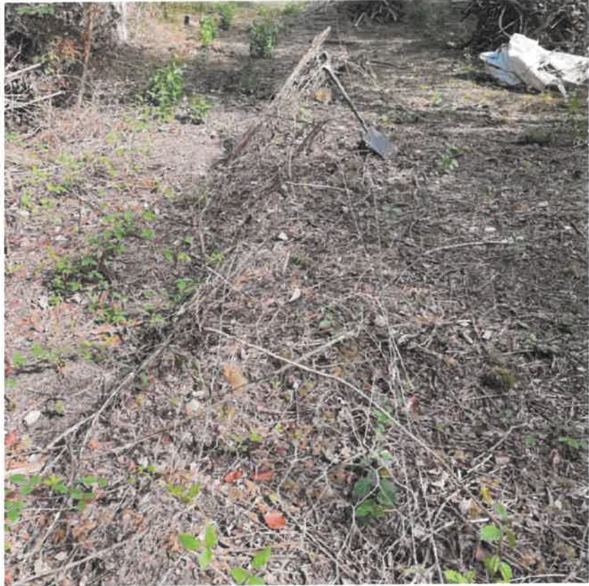
FENCE LINE CLEARED OF INVASIVE SCRUB TO ENABLE ACCESS FOR REPLACEMENT OF FENCE POSTS (20/8/23 WITH 1 METRE SPADE FOR SCALE)
