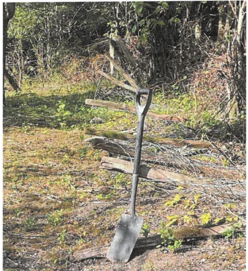
FENCE LINE CLEARED OF INVASIVE SCRUB TO ENABLE ACCESS FOR REPLACEMENT OF FENCE POSTS (20/8/23 WITH 1 METRE SPADE FOR SCALE)
