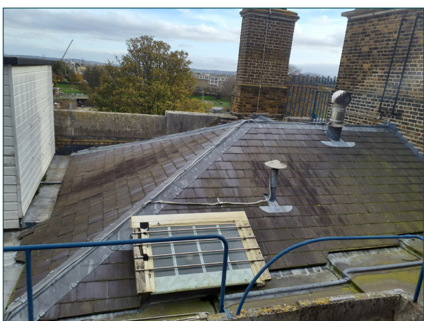
Photograph 5. Slate roof of B6
