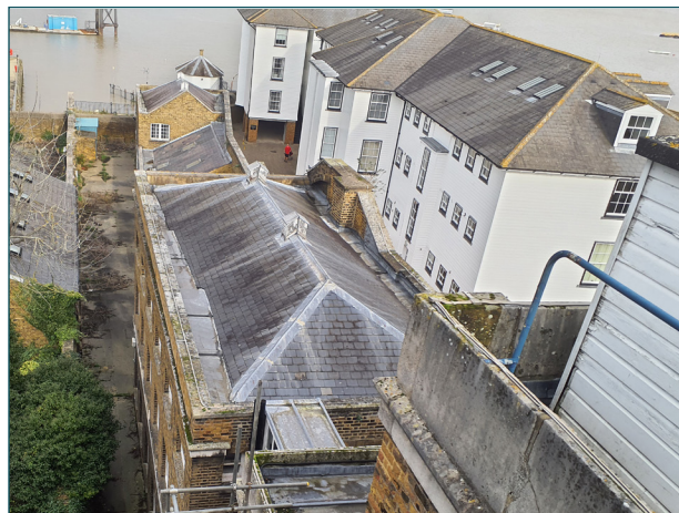
Photograph 4. Slate roof of B5
