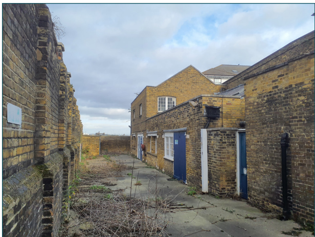
Photograph 3. West elevation of B5
