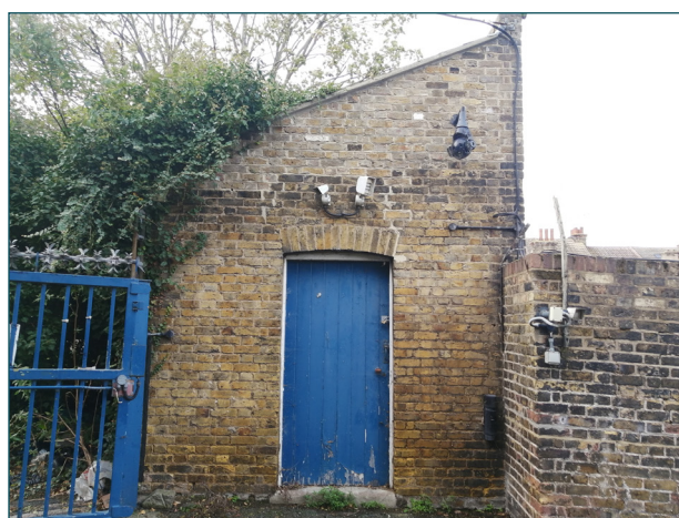
Photograph 6. South elevation of B7
