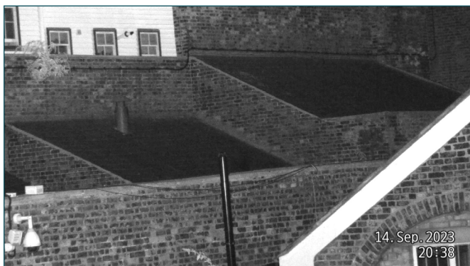
Photograph 1. NVA - Surveyor Location 2. Building B5
