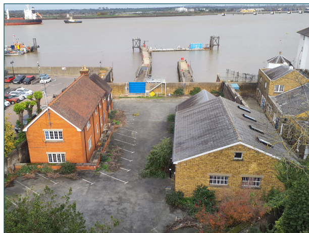
Photograph 2. B1 and B2 - showing well maintained roof tiles and slates
