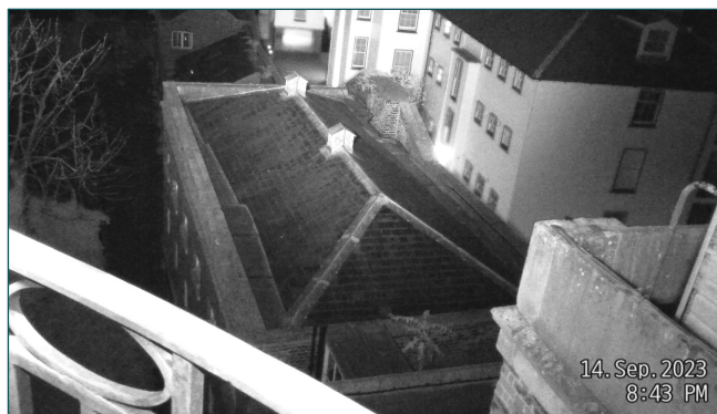
Photograph 2. NVA - Surveyor Location 6. Building B5
