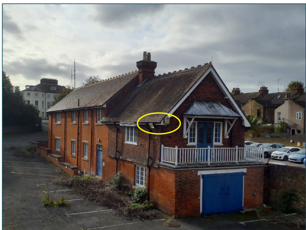
Photograph 1. Northern elevation of B1 showing location of security light
