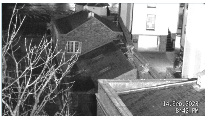
Photograph 3. NVA - Surveyor Location 7. Building B5
