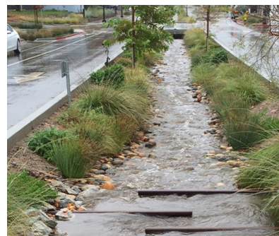
Wet ditch swale designed as barrier in conjunction with planting to prevent cats from migrating across site boundary into SSSI.
