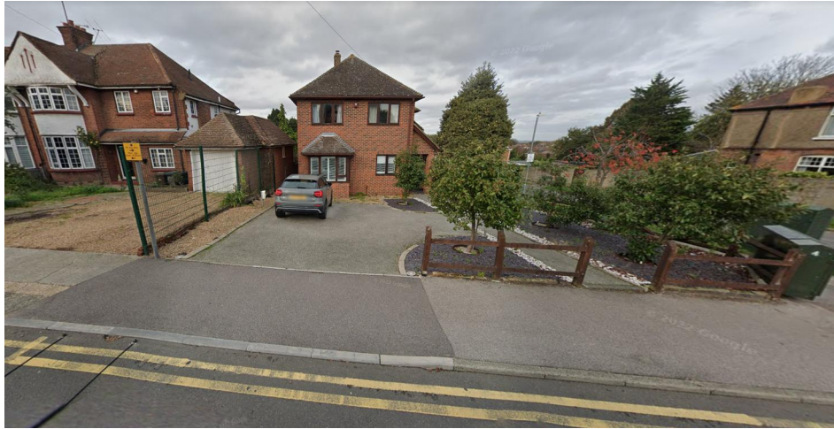
View of the permitted vehicle crossover 75 Old Road East.
