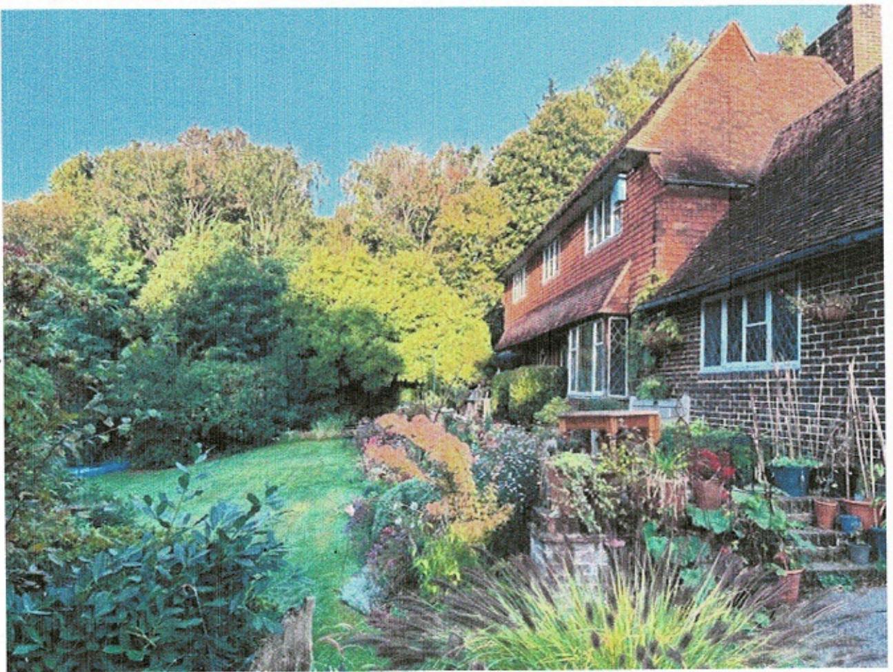
Photo 2. Note the first window (existing) which the bay will be extended from
