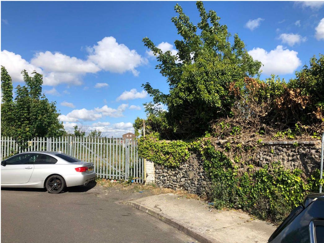
2. Edge of application site and the end of the flint wall
