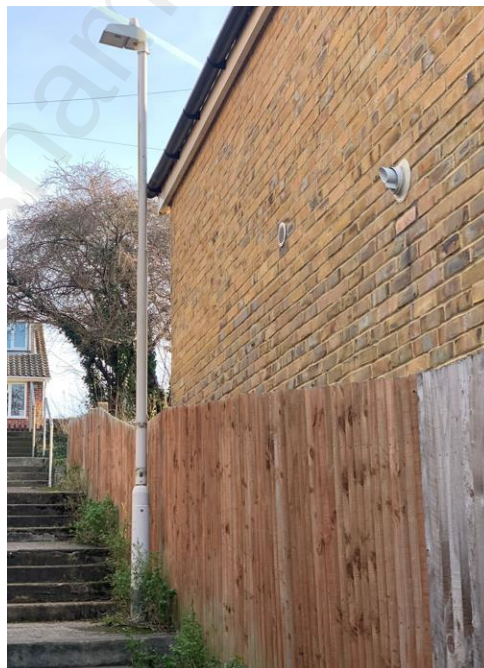
Photos of extension added to No. 43 Lyndhurst Way up to its side boundary with public footpath.
