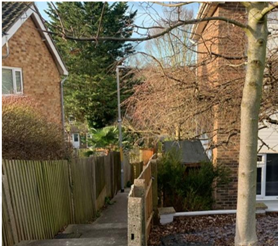
Views of front and rear of No. 25 Lyndhurst Way showing principal front and rear facing main windows serving ground floor space and only high-level secondary window on flank elevation with shed outbuilding positioned in front of it.
