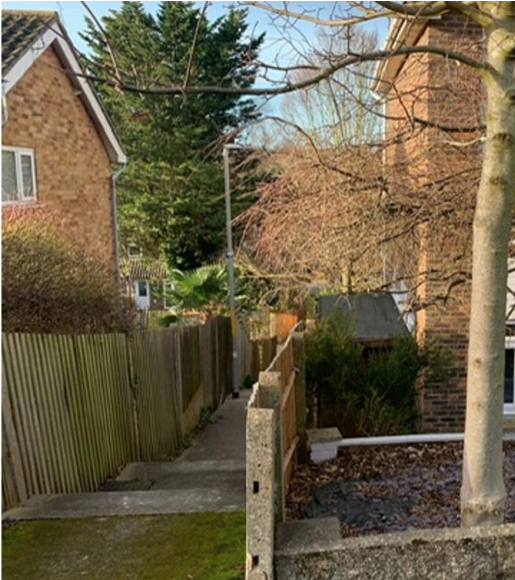
View showing street lighting serving public footpath
