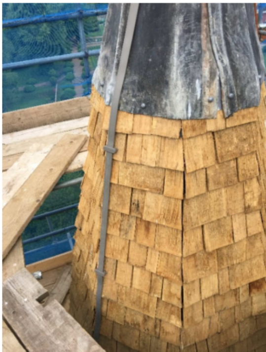
Oak shakes as laid new at another Kent church summer 2018
