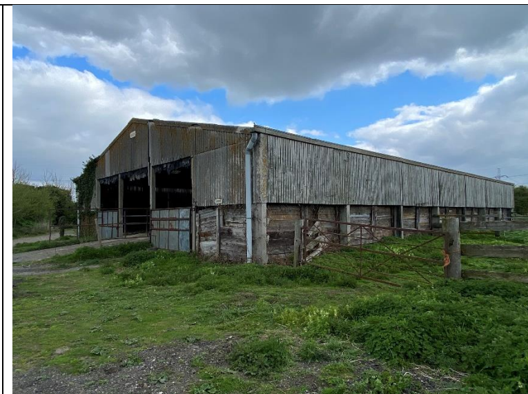
Figure 1 Southern and western elevation of B1.
