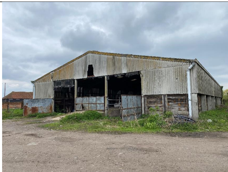
Figure 2 Eastern and northern elevation of B1.
