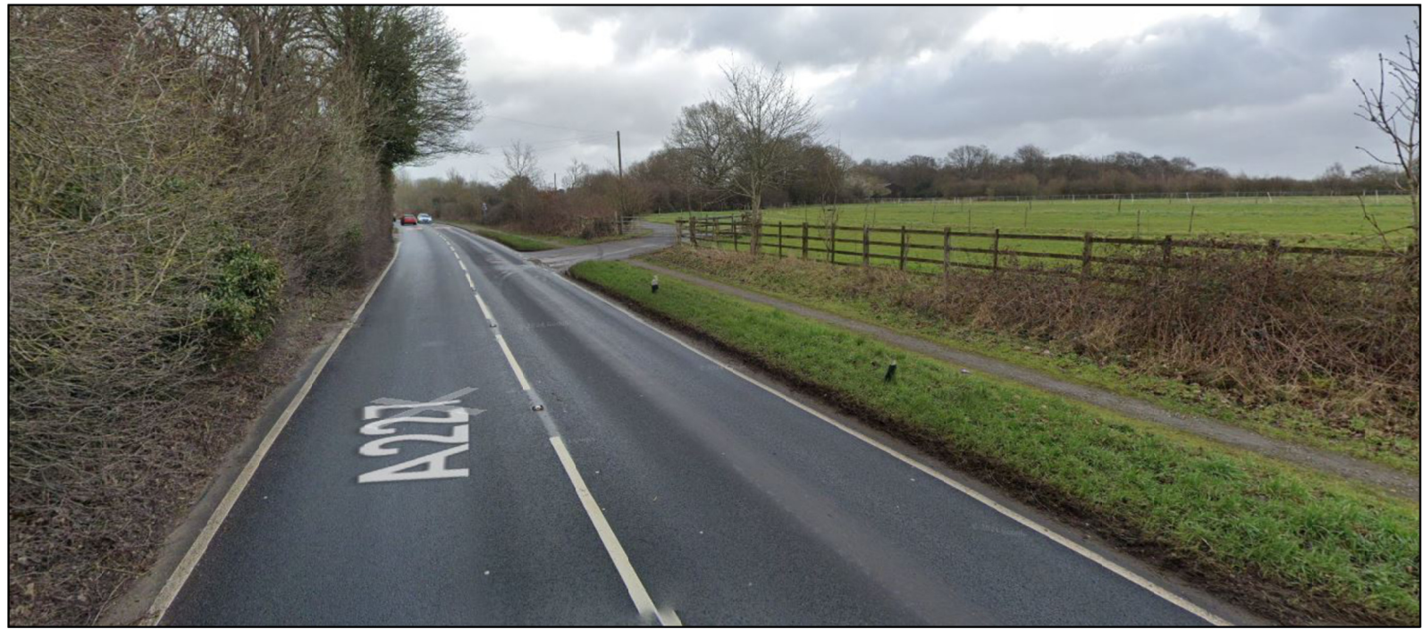
Image of Existing Access showing suitable unobstructed splays already in existence.
