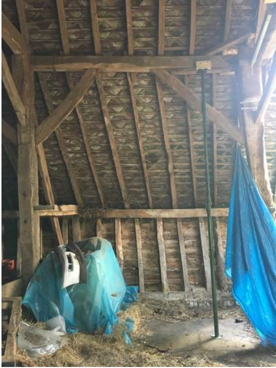
Fig 15. Bay 4 - South aisle
