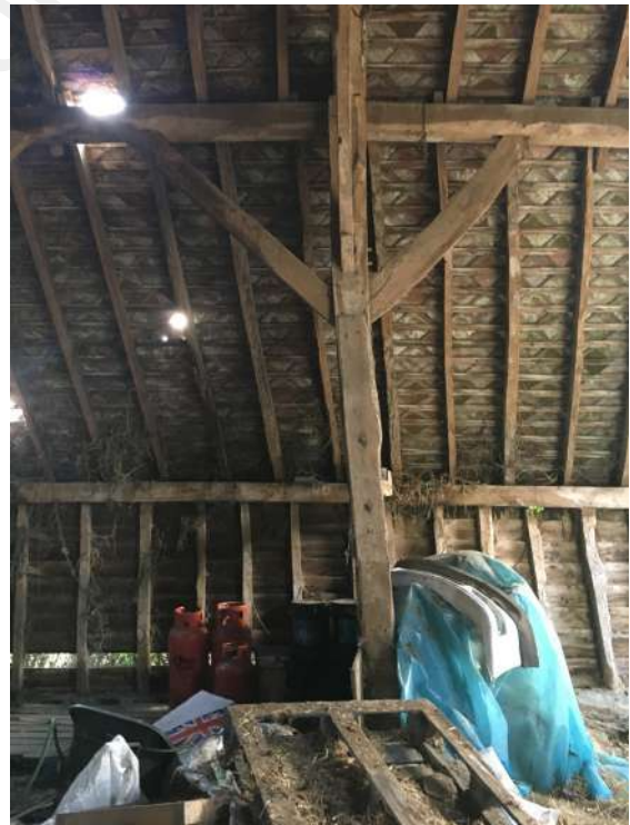
Fig 17. Bay 3 - Temporary repairs to main tie beam
