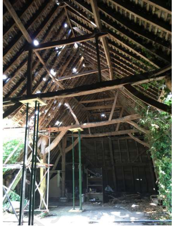
Fig 16. Bay 4 - Looking towards bay 1-3
