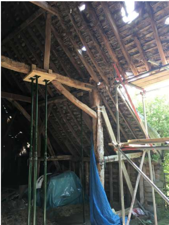
Fig 17. Bay 3 - Temporary repairs to main tie beam
