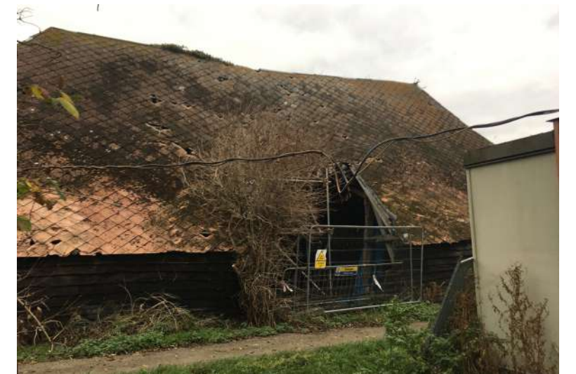
Kent barn south east elevation in winter
