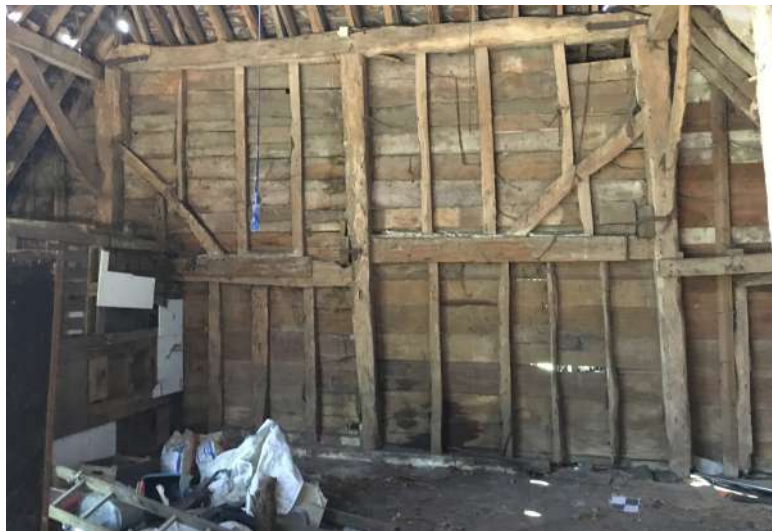
Kent barn - Internal framing
