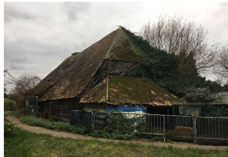
North east corner of Kent barn in winter
