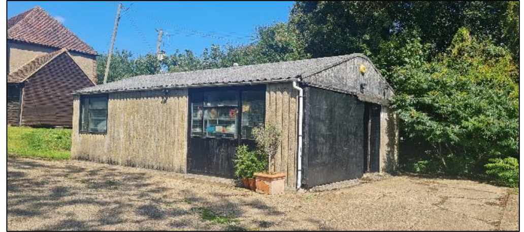
Picture 1: Looking north-west at the eastern and southern elevations of B1.
