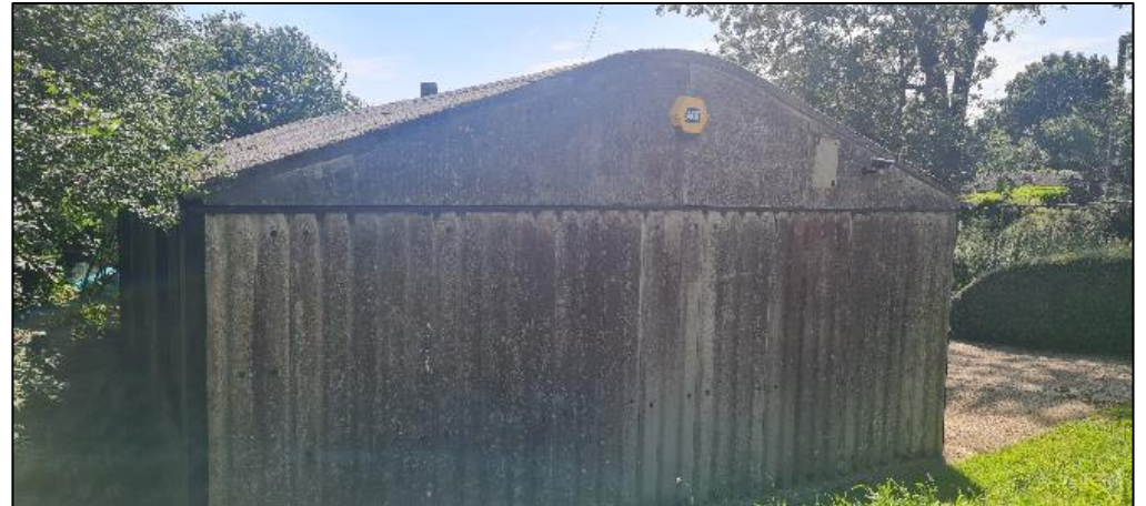
Picture 2: Looking south-east at the northern and western elevations of B1.
