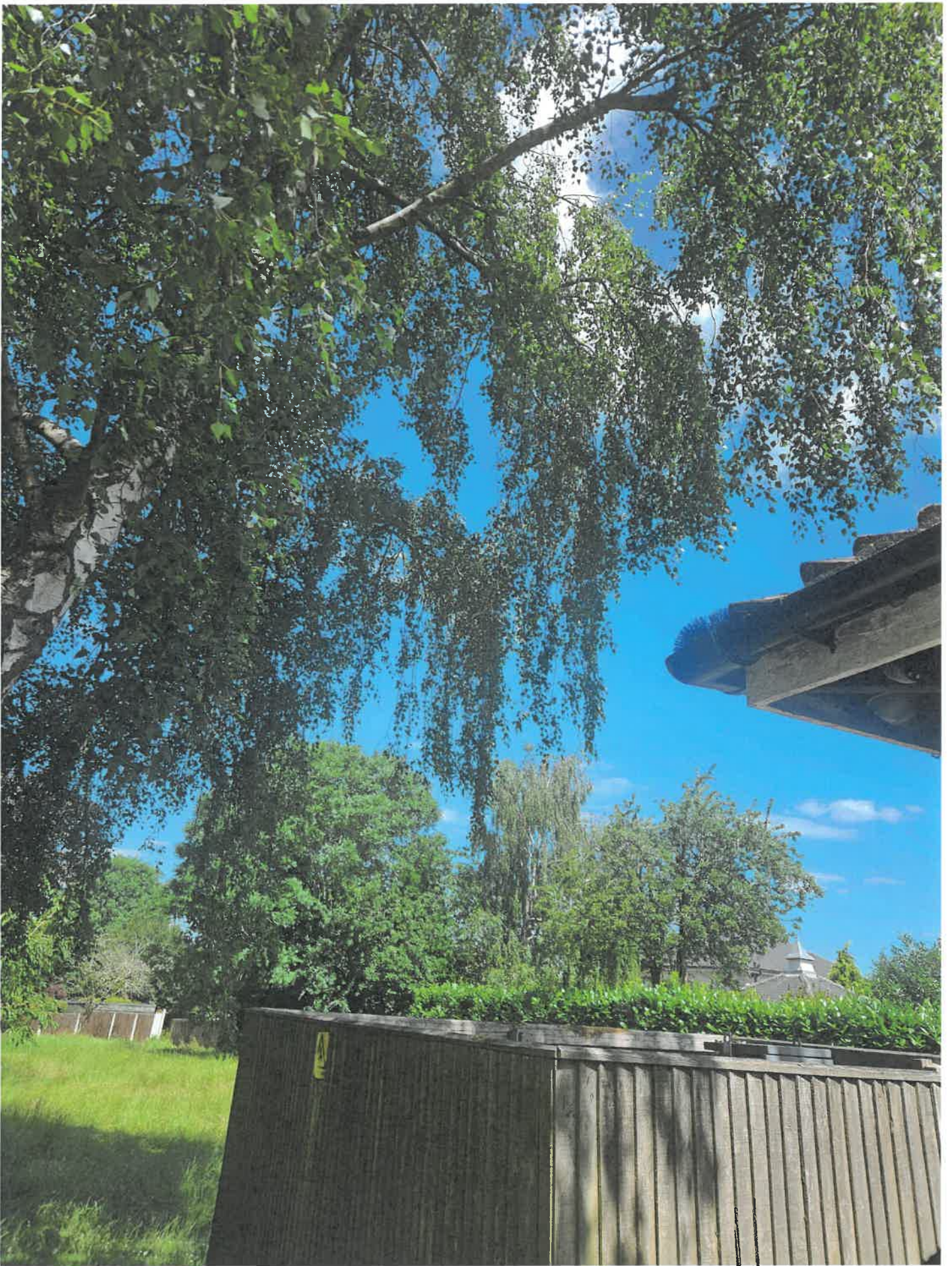
⑤ SILVER BIRCH - OVERHANGING ELECTRICAL SUB STATION - REQUIRE CROWN LIFT.
