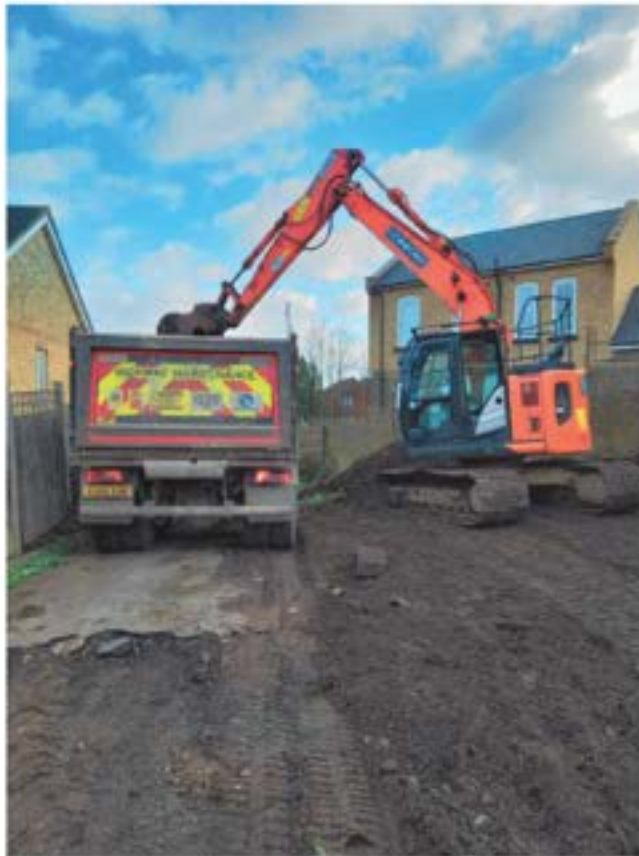
Photo 8 - Lorry and mechanical excavator used to remove coal tar rich tarmac
