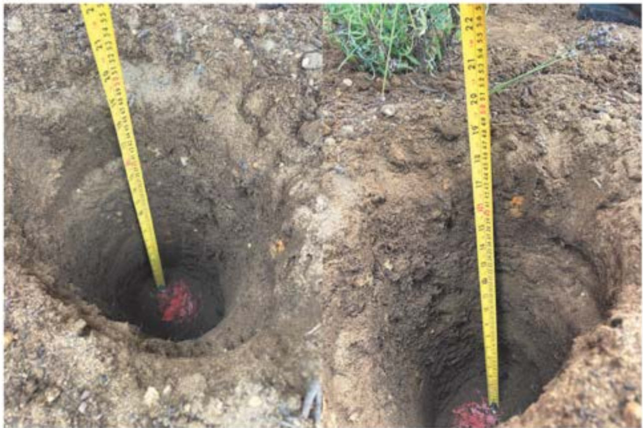
Photos 14, 15 + 16 - Examples identifying the depth of ground removed to afford clean cover system and hi-visibility membrane
