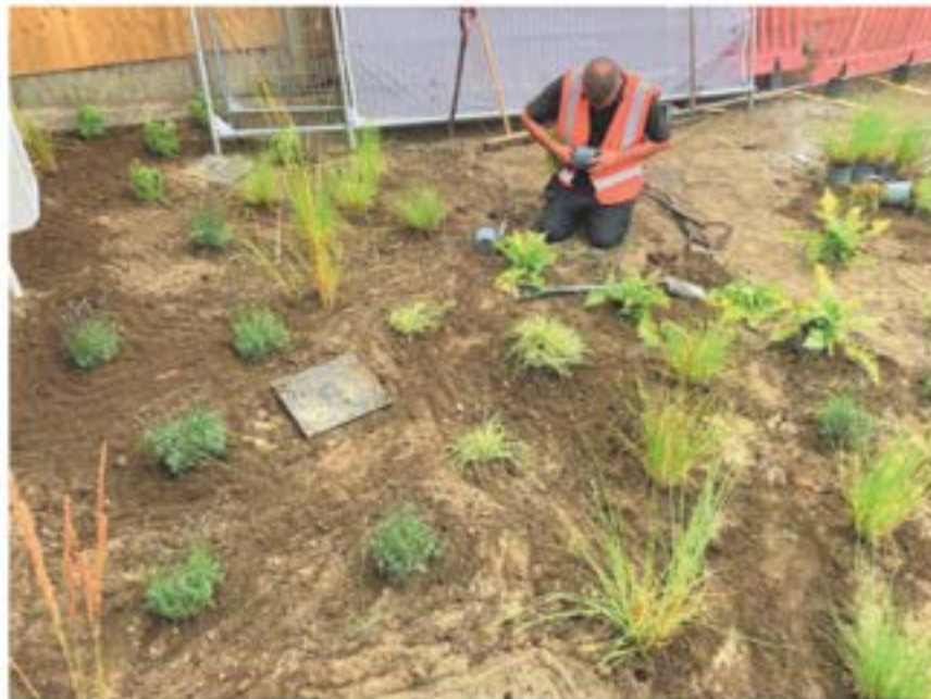
Photo 24 - Example reinstatement of soft landscaping
