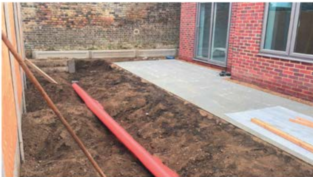
Photo 27 - Example of hi-visibility geotextile membrane used
