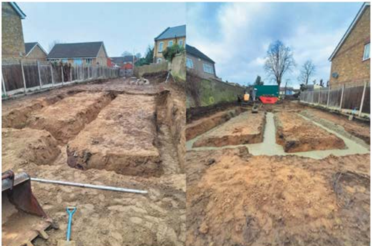
Photos 12 + 13 - Examples of trenches dug for foundations
