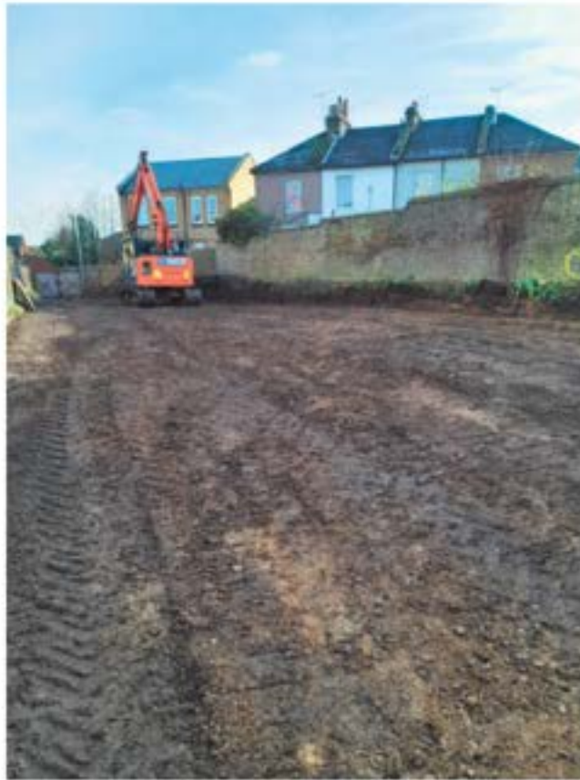
Photo 11 - Example photo showing levelled site
