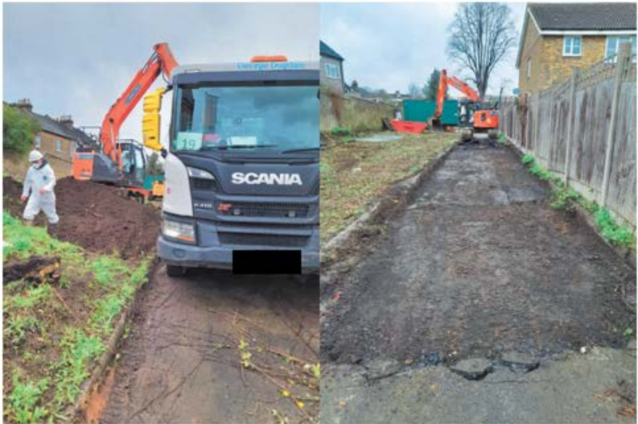
Photos 1 + 2 - Showing area of remedial excavation for asbestos testing, identifying PPE, mechanical excavator and lorry for disposal
