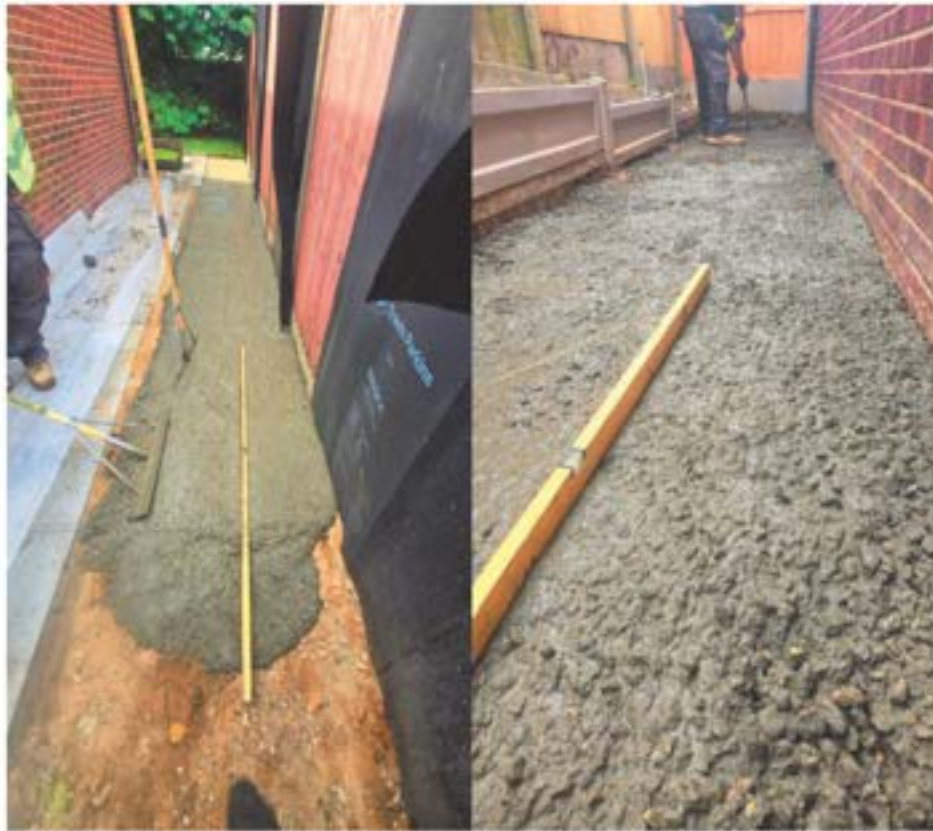
Photos 22 + 23 - Examples of reinstatement with concrete hardstanding
