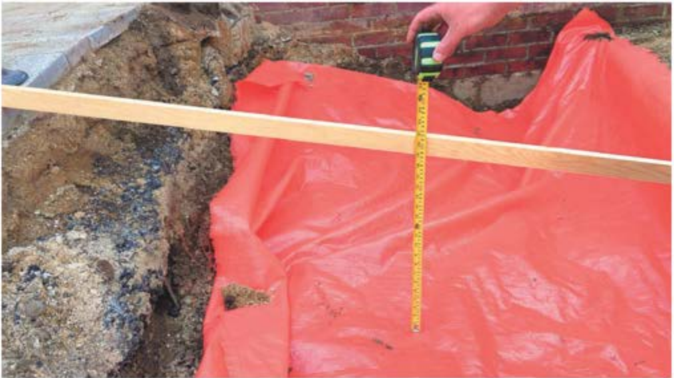
Photos 14, 15 + 16 - Examples identifying the depth of ground removed to afford clean cover system and hi-visibility membrane
