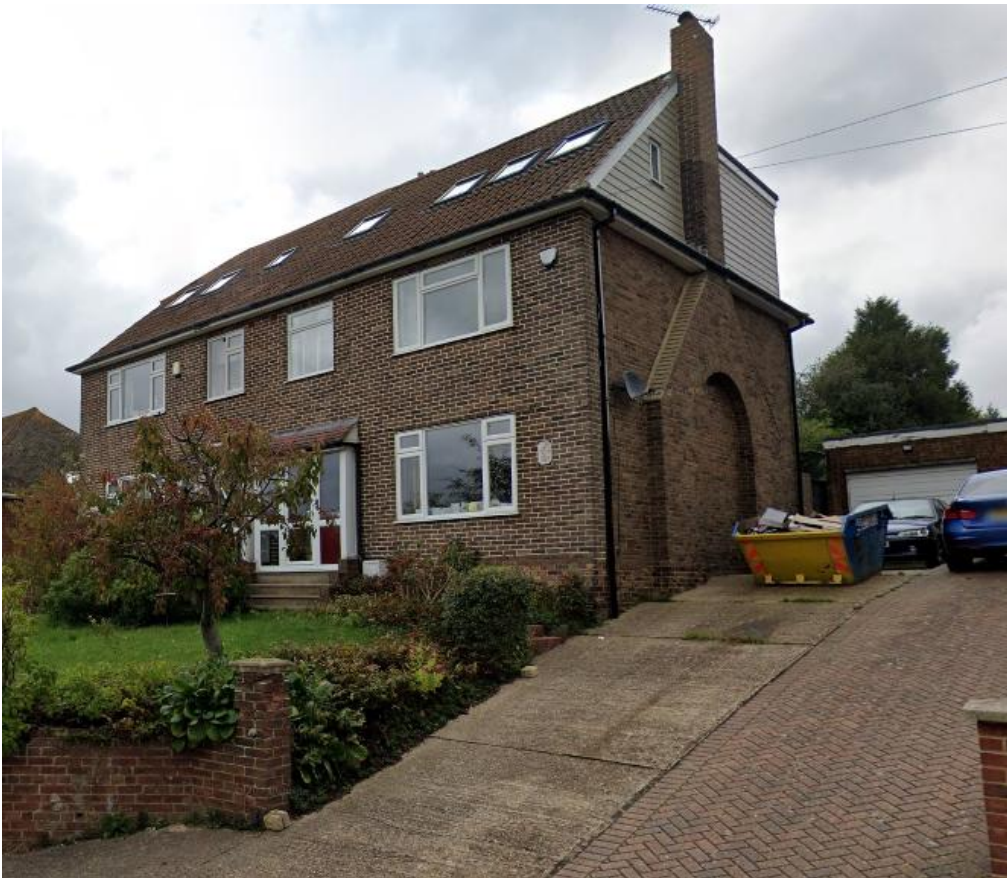
Closer view of the side of no. 383 showing the gable roof extension and rear dormer extension
