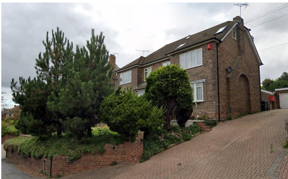
Closer view of adjacent semi-detached dwelling no. 387 Valley Drive with a half hip roof extension
