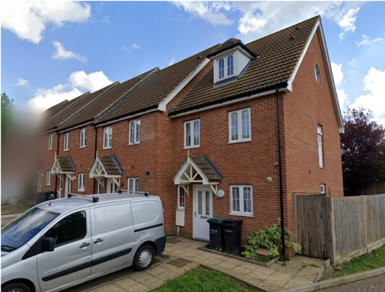
Original Photograph of the site
