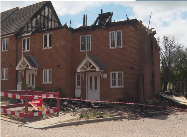
Existing Photograph of the site
