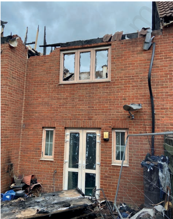
Fig 8 Existing Rear Elevation to No. 108.
