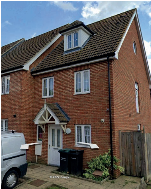
Fig 3 Original Front Elevation of No. 104.
