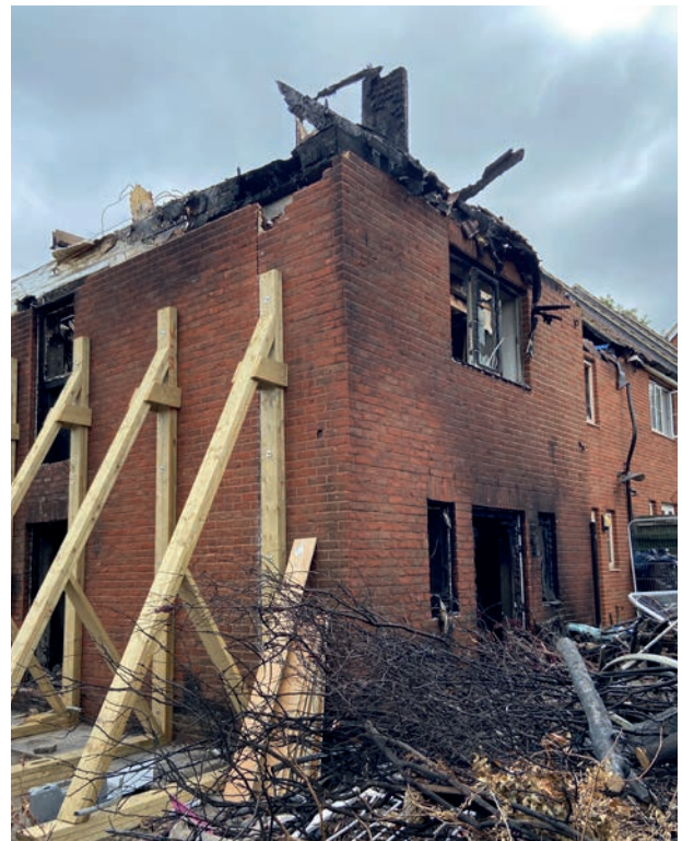
Fig 9 Existing Rear Elevation to No. 104
