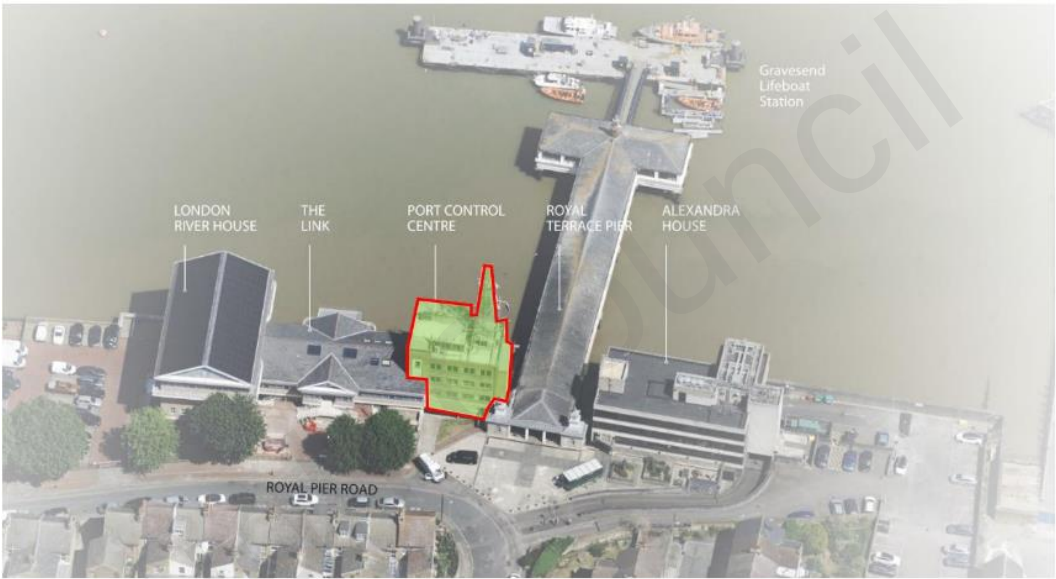
Figure 2 Port Control Centre Building for Proposed Refurbishment
