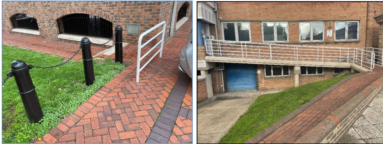
Figure 6: Existing black bollards outside London River House and white fencing proposed to be removed
