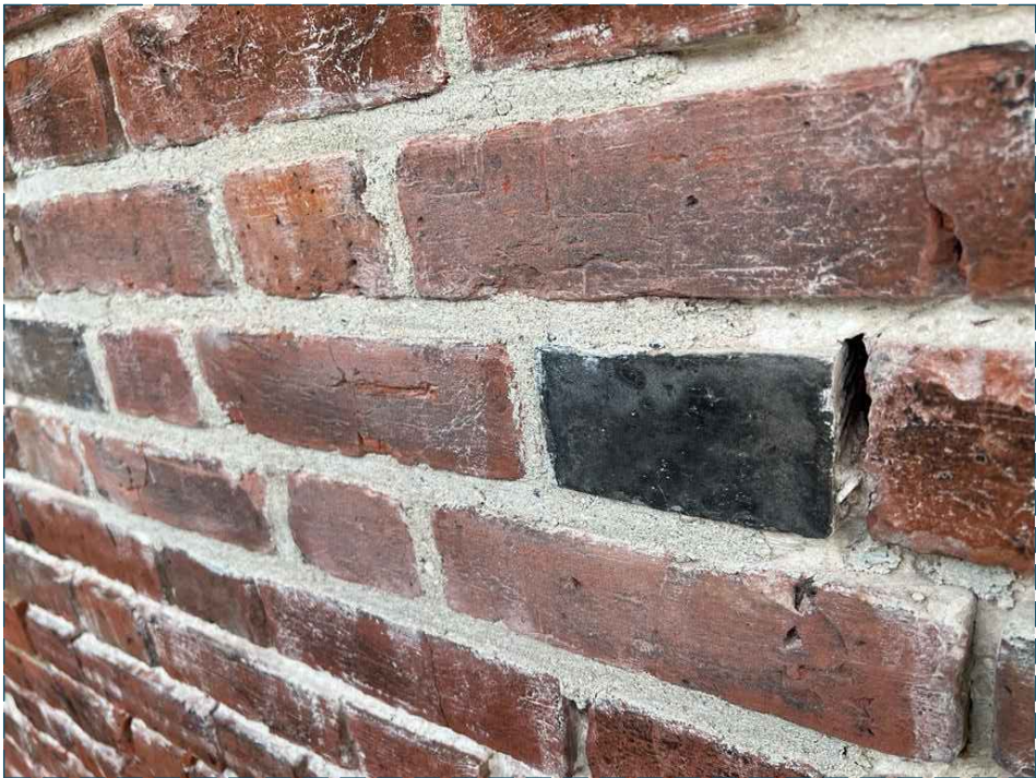
PIC 03 SAMPLE PANEL PRODUCE IN MARCH 2023 AND TO BE USED AS REFERENCE FOR REPOINTING.
