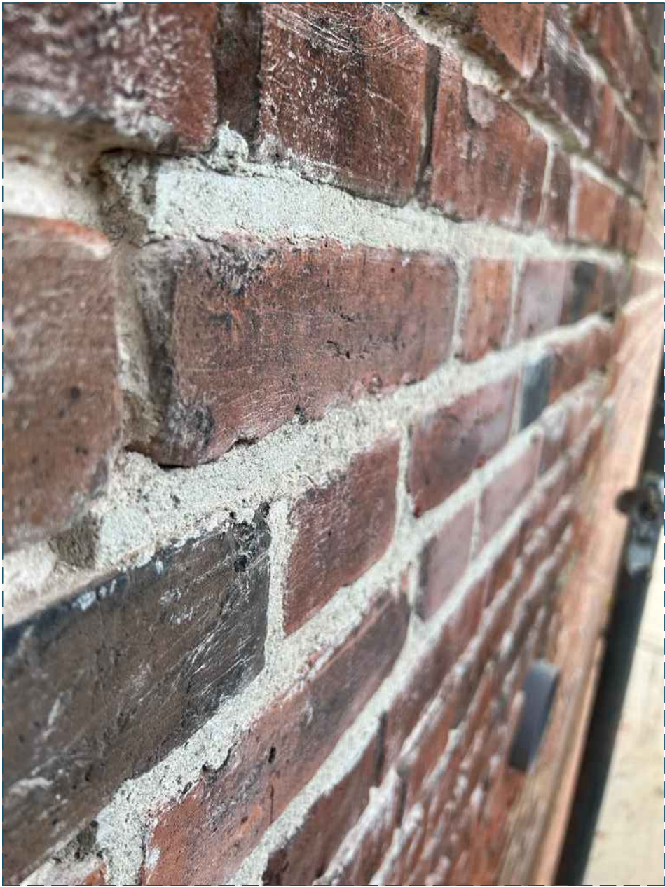
PIC 02 SAMPLE PANEL PRODUCE IN MARCH 2023 AND TO BE USED AS REFERENCE FOR REPOINTING.
