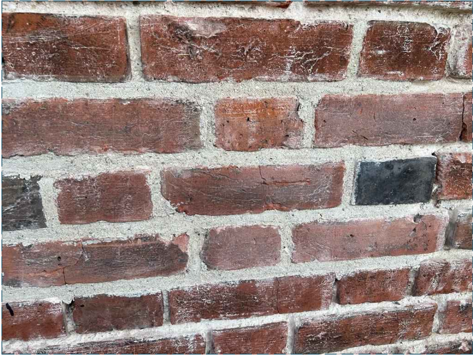
PIC 01 SAMPLE PANEL PRODUCE IN MARCH 2023 AND TO BE USED AS REFERENCE FOR REPOINTING.
