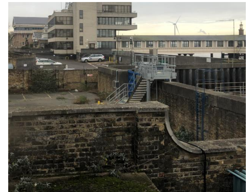
Photograph showing Sea Defence wall with blue flood gate and access stairs visible.
