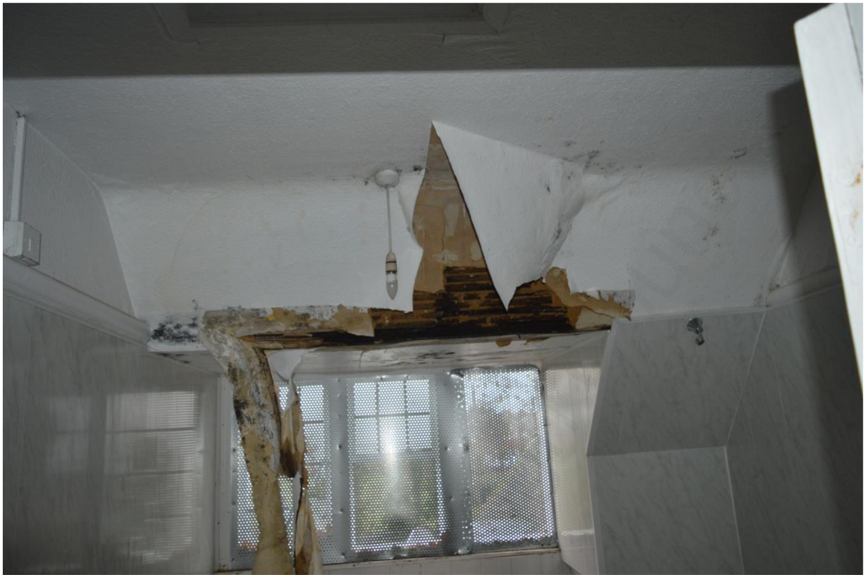
Photograph 8: Internal damage to the ceiling (downstairs)
