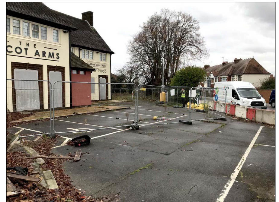
21. Proposed development area. Existing frontage parking area. Facing NW, Ascot Road to R
