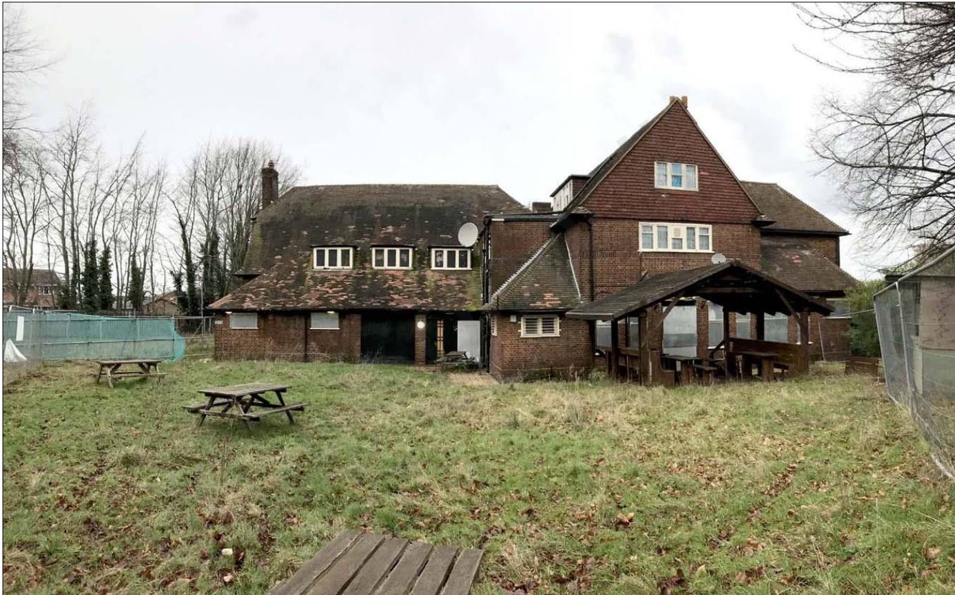
14. Proposed development area. Rear of the existing building and garden, facing NW
