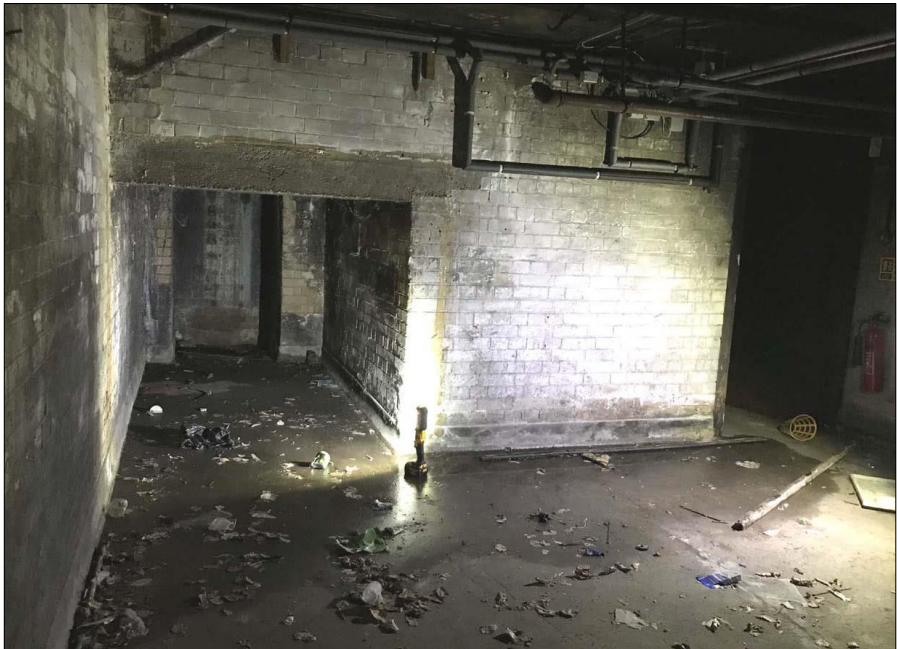
27. Basement/ boiler room. Facing W
