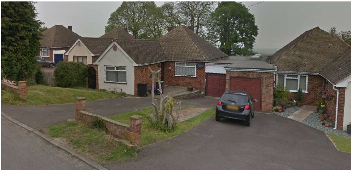
Front No 20, showing Nos 18 (right) and 22 (left)
