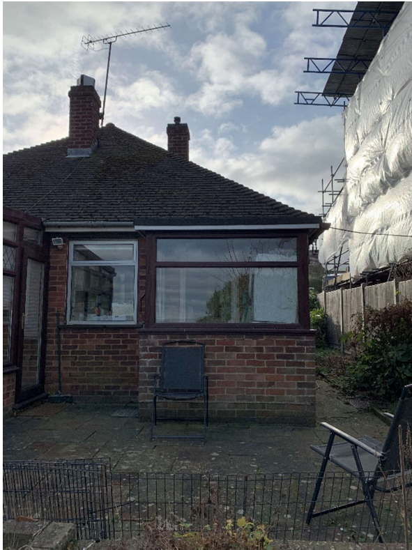
Rear No 20 Looking towards No 22
