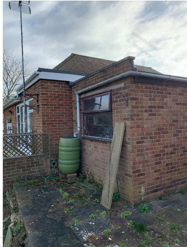
Rear No 20 garage Looking towards No 18
