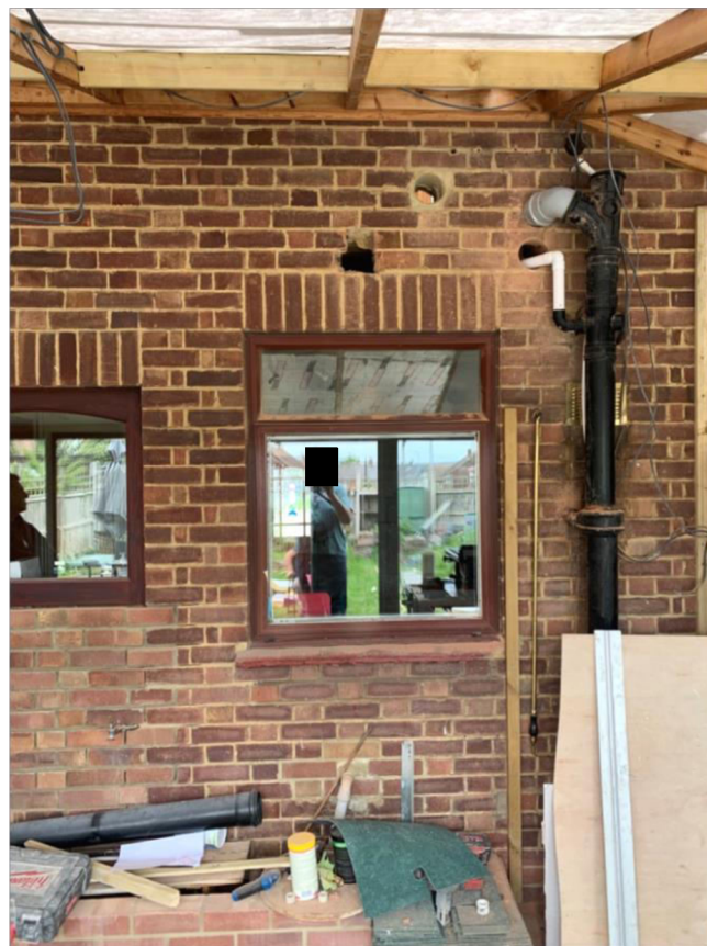
Existing Kitchen windows
