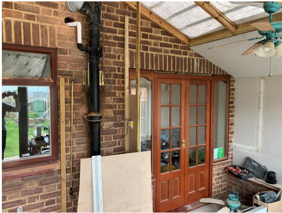
Existing double door to rear of existing lounge/dining
