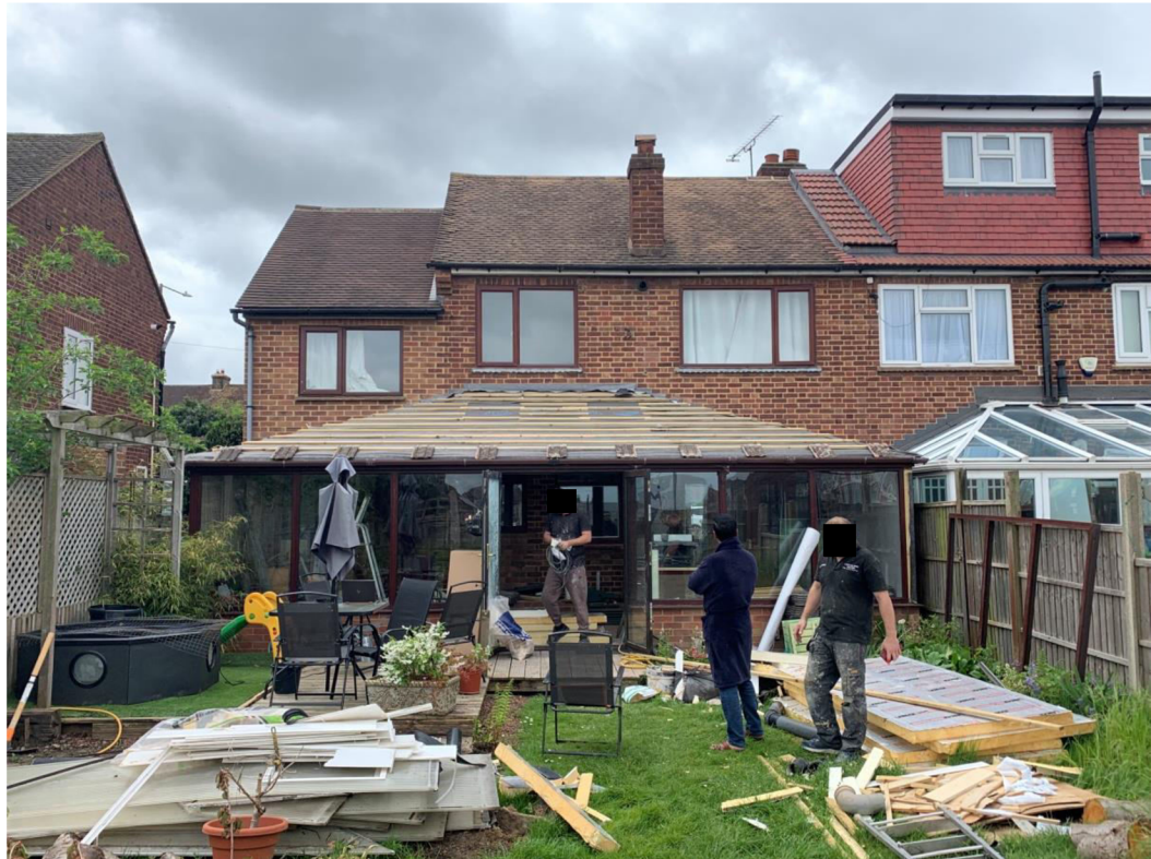
North Elevation as seen from the back garden
