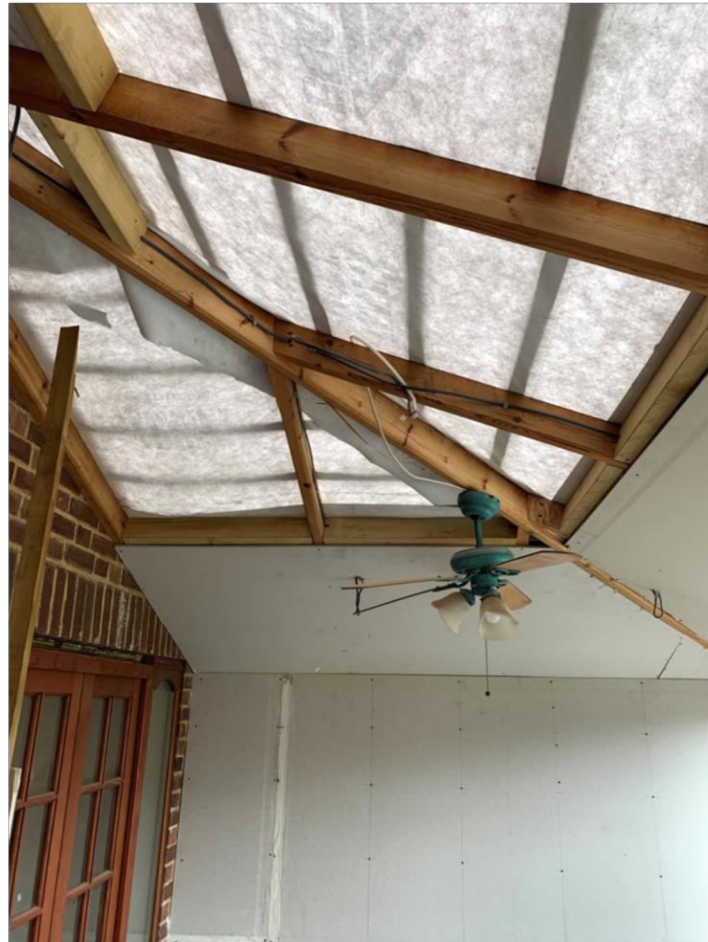
New Insulation to Conservatory Ceiling
