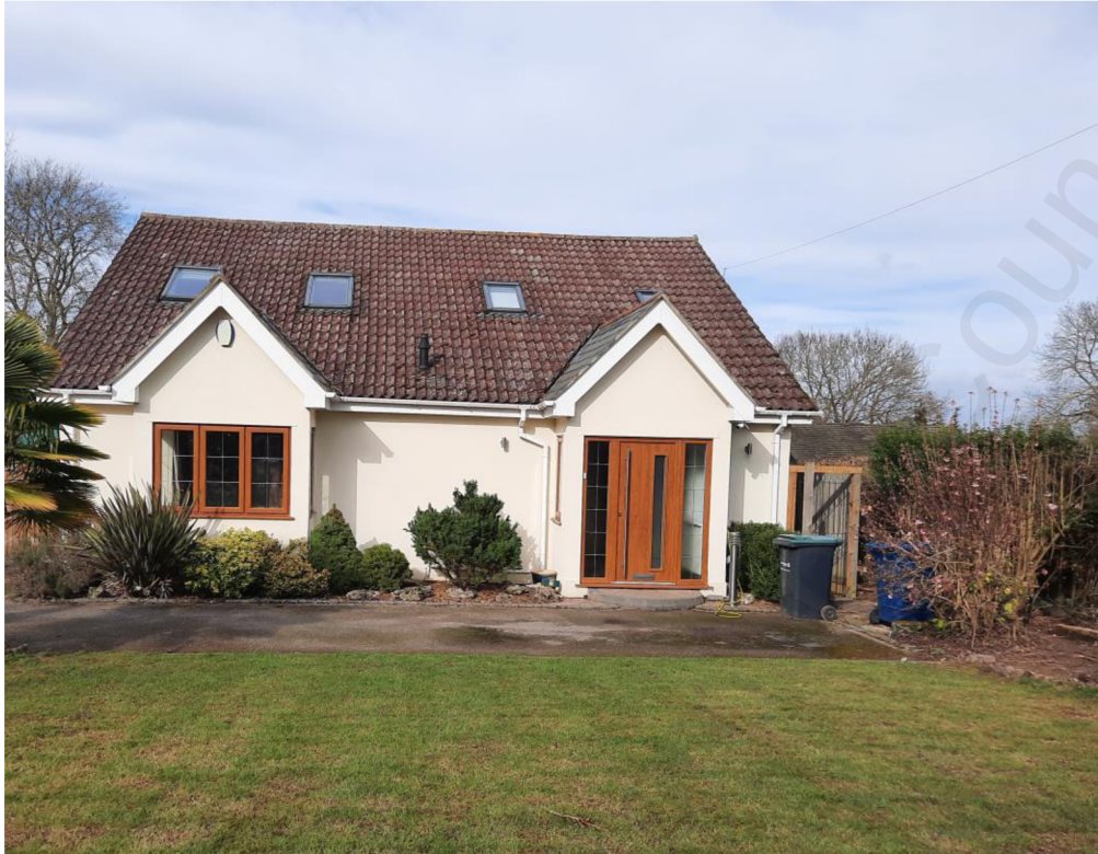
Photograph B: The rear elevation
