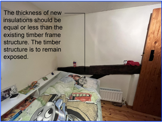
First Floor Bedroom
