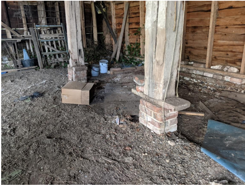
Photograph 13 - Internal brick plinths
