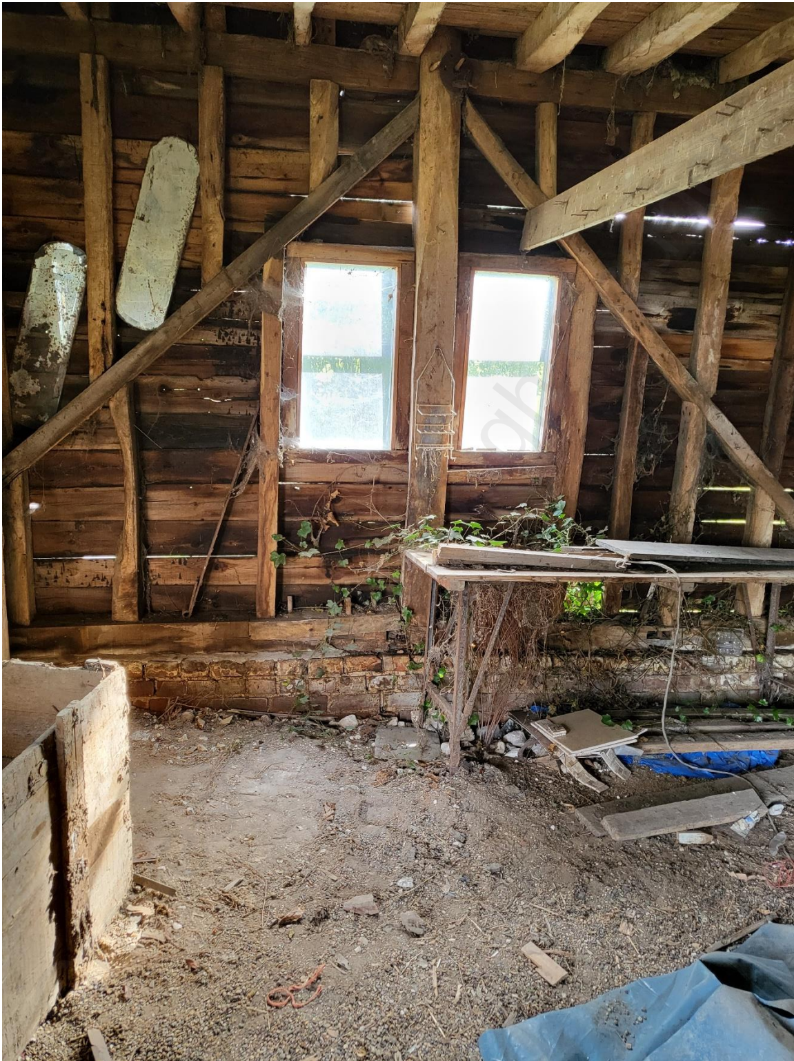
Photograph 18 - Window and framing around south window
