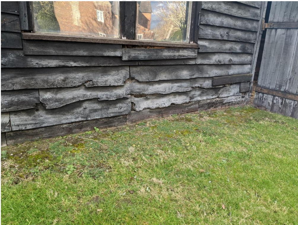
Photograph 16 - Weather boarding to east elevation
