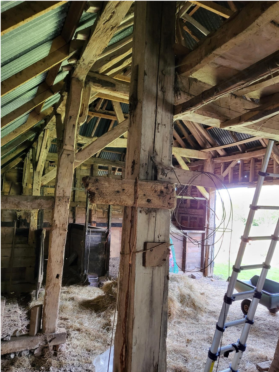
Photograph 1 - Brace beams to West Elevation
