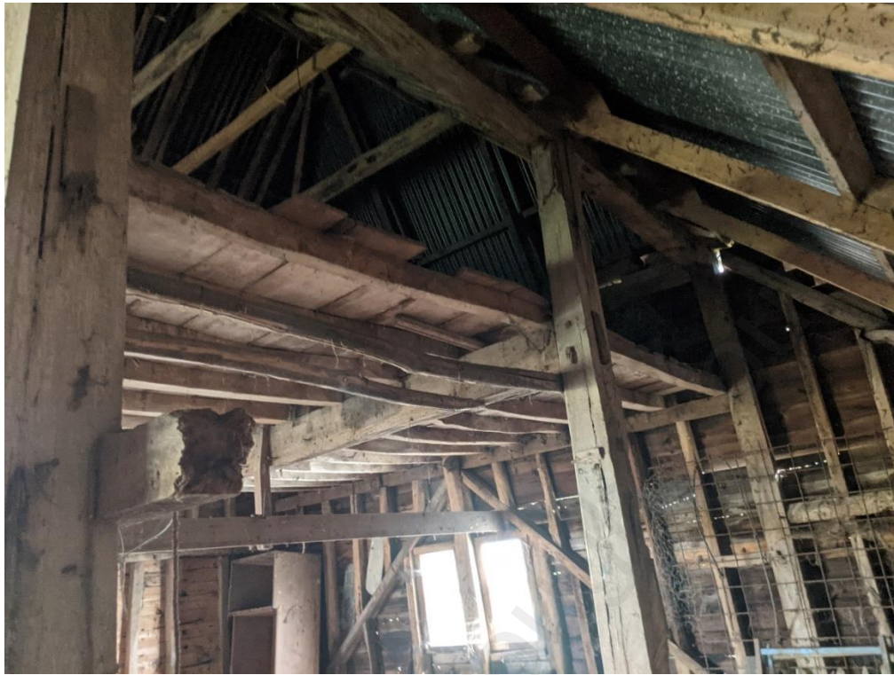
Photograph 11 - Shallow floor joists to mezzanine
