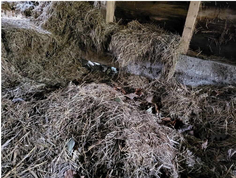
Photograph 22 - Concrete edging to sole plate in north stable
