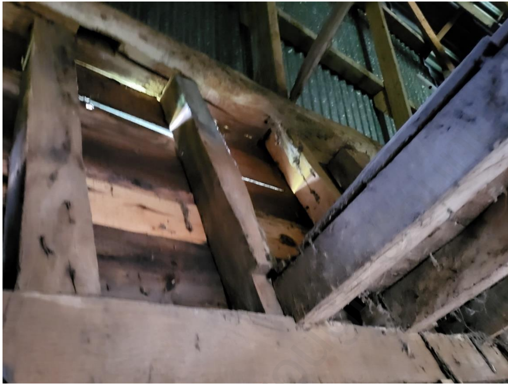
Photograph 19 - First floor joist bearing to south wall
