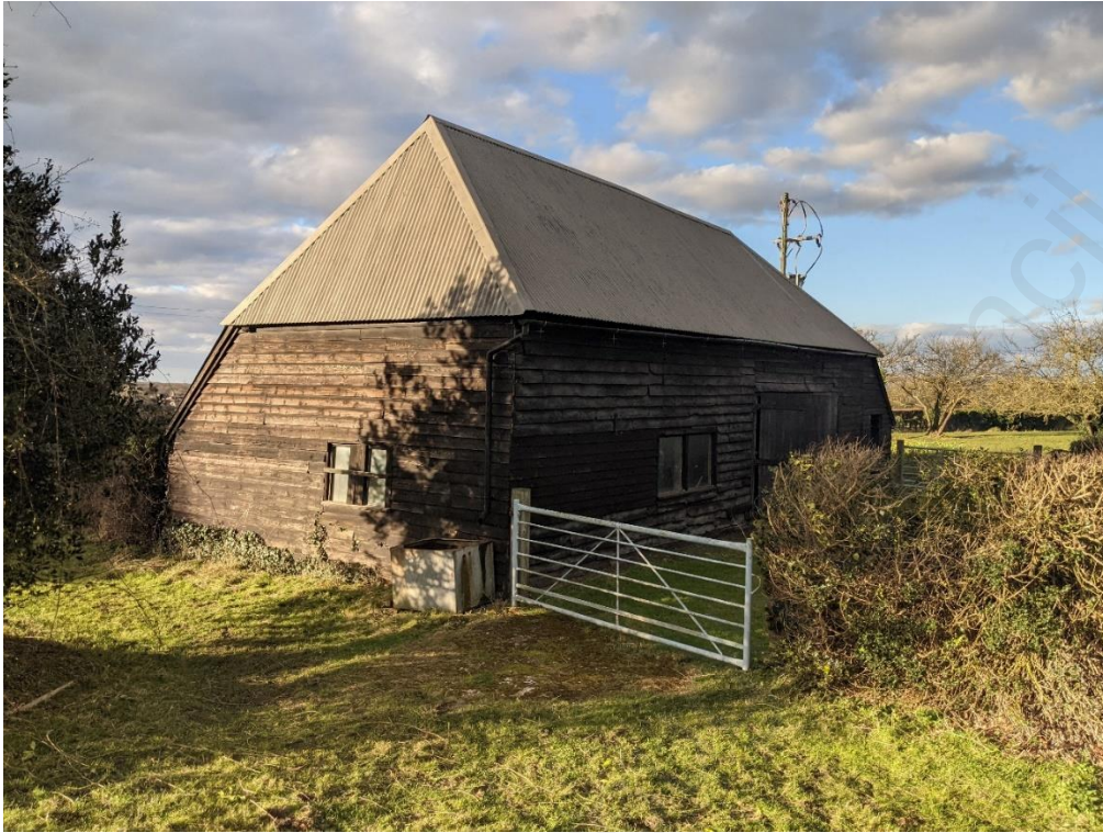
Photograph 15 - External roof cladding to barn
