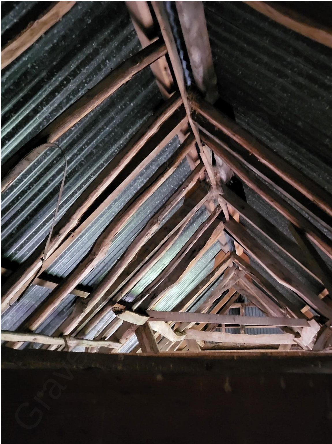
Photograph 10 - Ridgeboard insert to roof and new rafters
