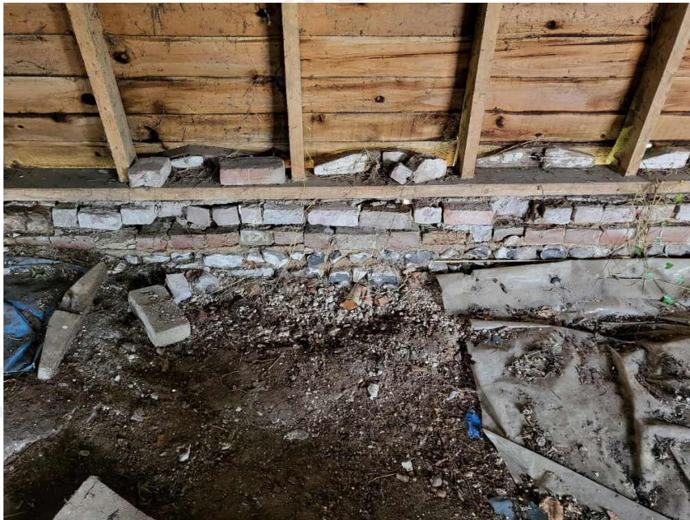
Photograph 14 - External plinth to west wall
