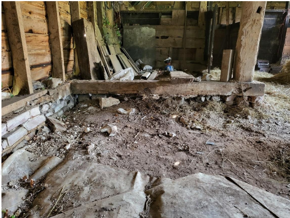
Photograph 12 - Internal plinth support inner post
