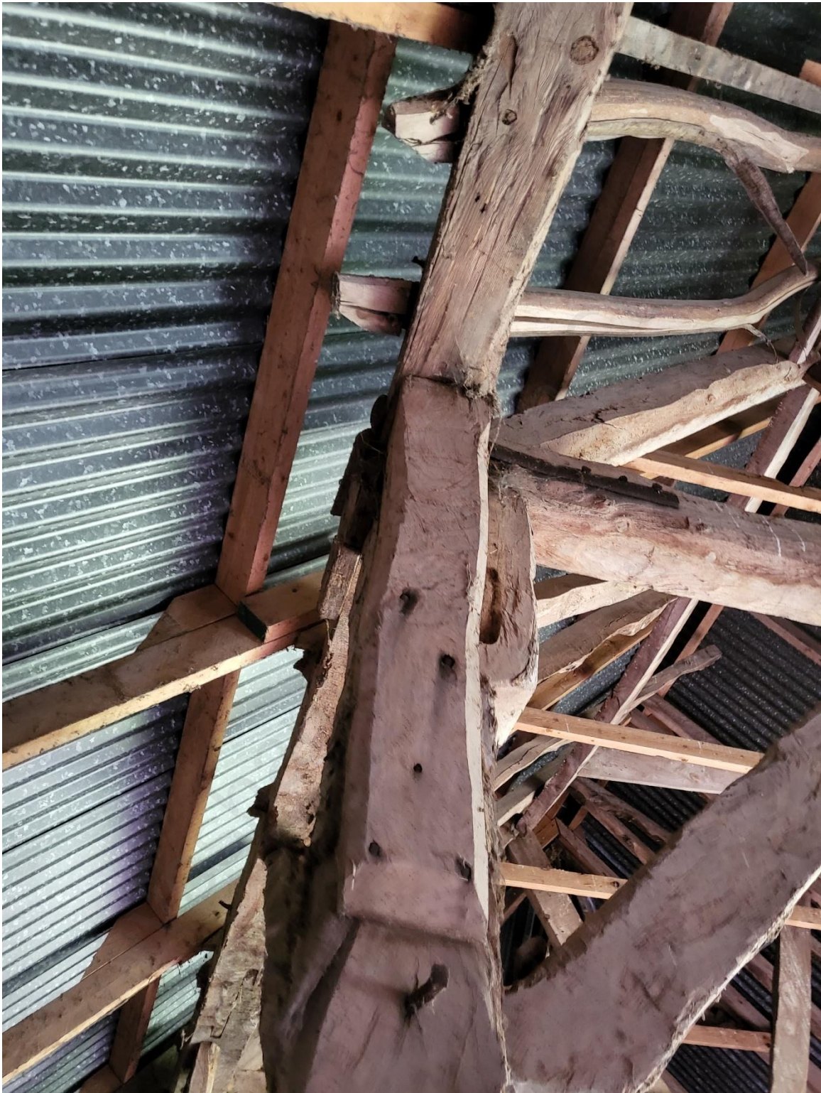
Photograph 20 - Strapping around eaves frame - grid 4
