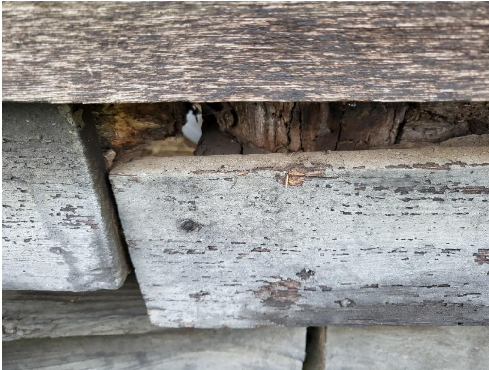
Photograph 6 - External face of window post on east elevation
