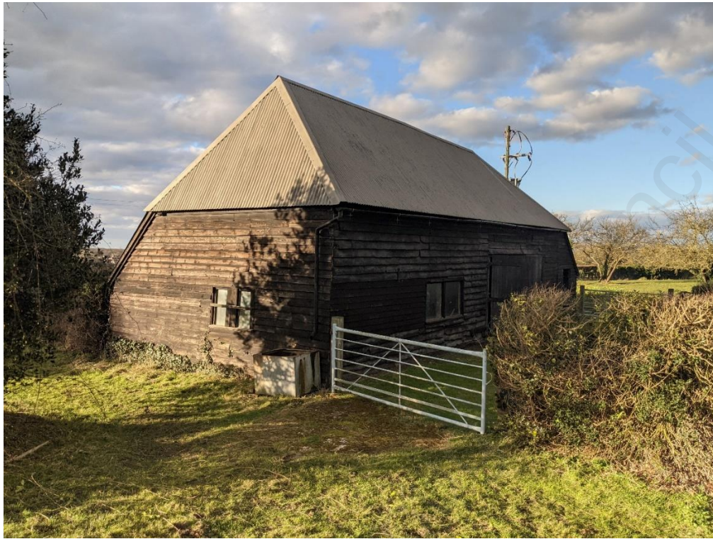
Photograph 15 - External roof cladding to barn
