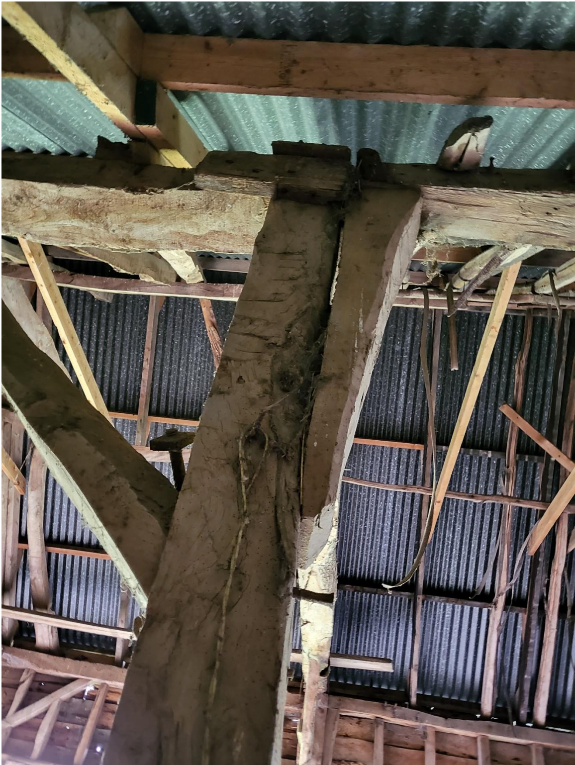
Photograph 4 - Side jowl fixings prising out
