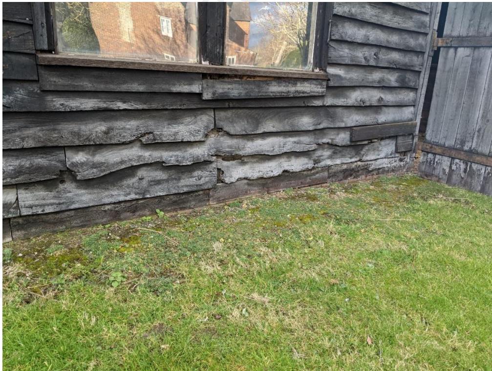
Photograph 16 - Weather boarding to east elevation
