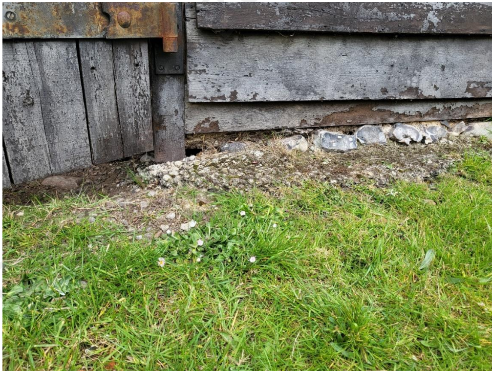
Photograph 7 - External sole plate with rot at ends
