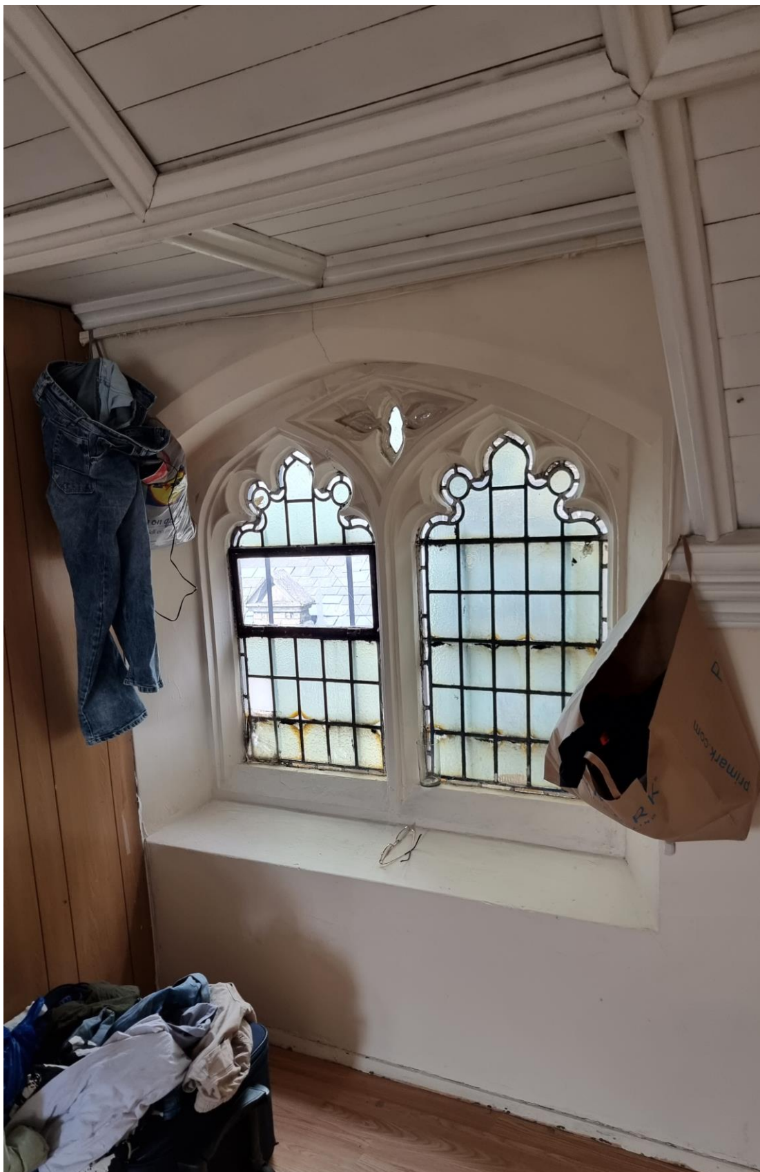
Fig.12: The former balcony to the chapel, now the mezzanine bedroom (room 25) with tracery window, barrel vaulted ceiling, and modern partition wall (left) to form the room.
