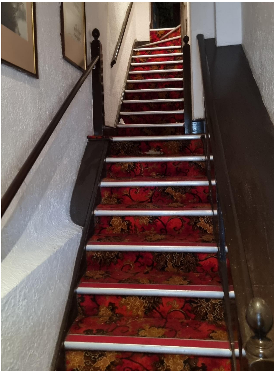
Fig.5: The stairs from the ground floor front entrance to the first floor. The lower section dates to c.1952 as part of the works to convert the ground floor to shops. The upper section is thought to be in its original position but altered around the same time.
