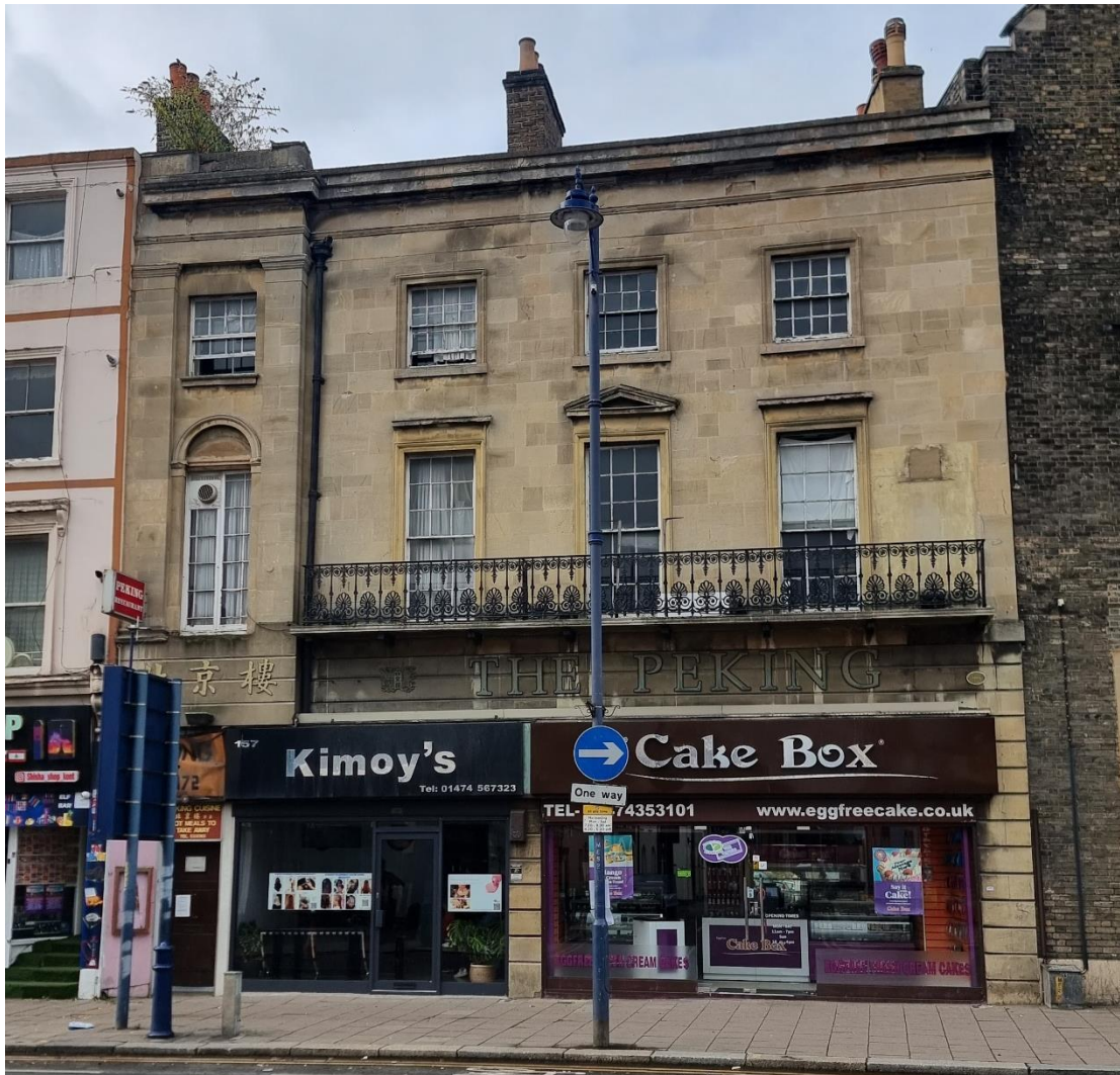
Fig.3: The principal north elevation of the property, seen from Milton Road.
