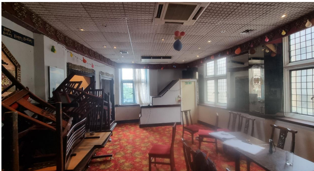
Fig.6: The first floor restaurant seating area to the rear of the buildings (room 7 of fabric assessment, HS3 ) which includes incongruous modern enclosed stairs to the ground floor.
