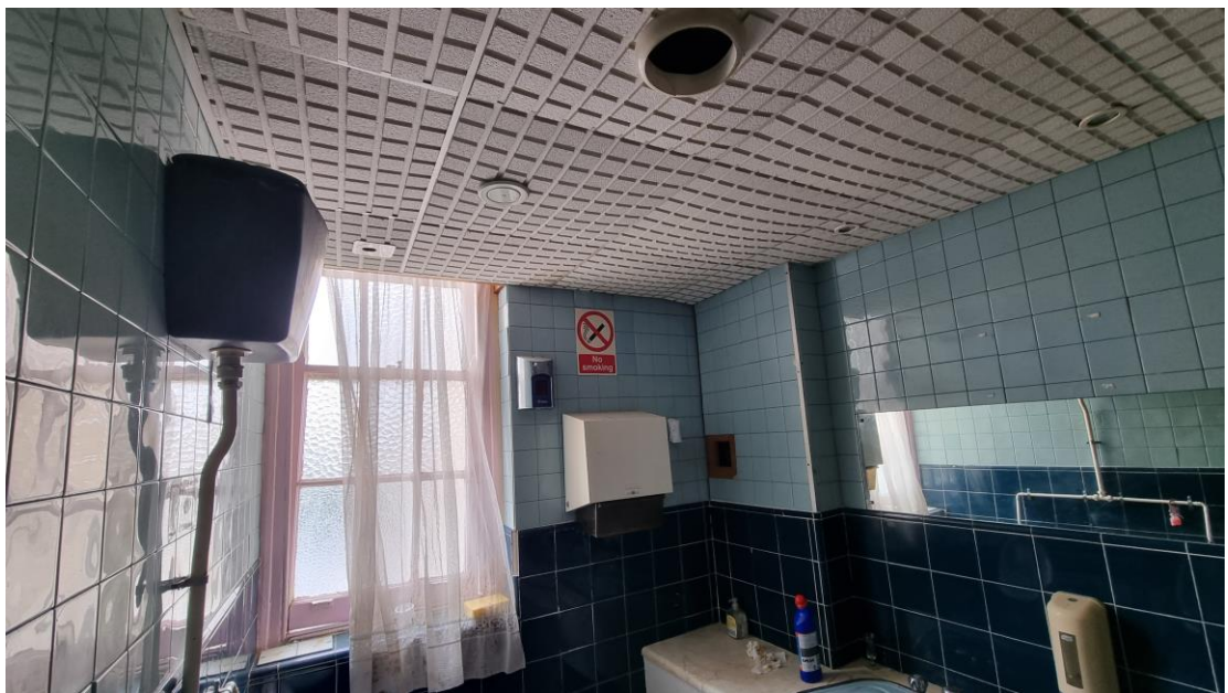
Fig.10: Modern first floor toilets (room 6).
