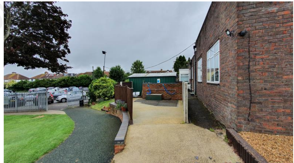
Fig 19—View of side compound
