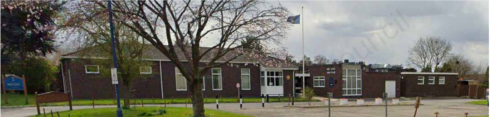
Club House from north, Singlewell Road
