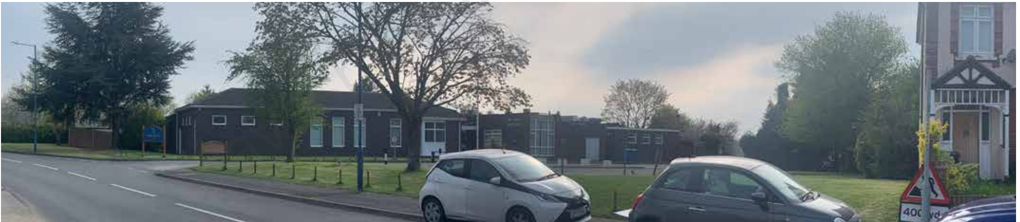
Site entrance viewed from north, Singlewell Road
