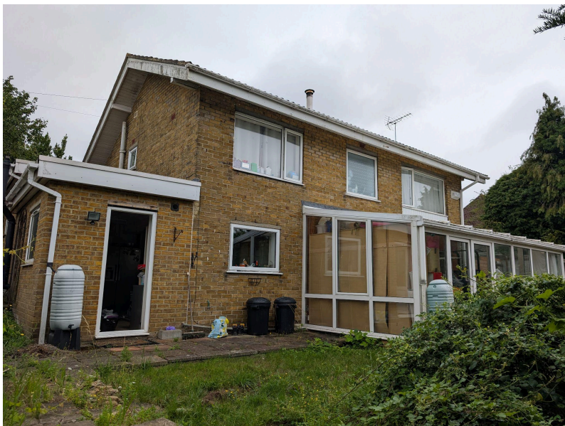
Existing rear elevation of the property
