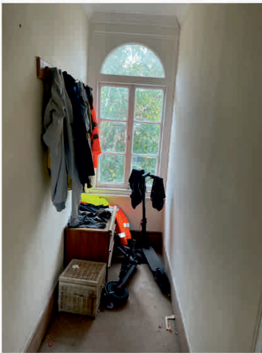
PHOTOGRAPH 6 Landing window at first floor being an intact original photograph it also illustrates the existing skirtings which are generally intact throughout
