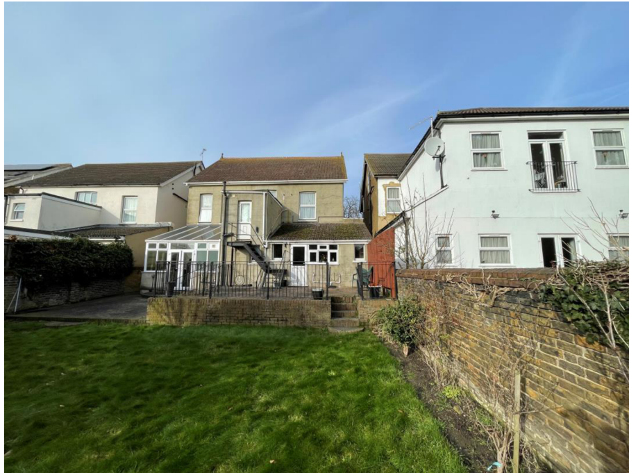
Fig 2 – Rear of No.54 Pelham Road
