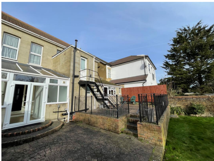
Fig 3 – Rear of No.54 Pelham Road
