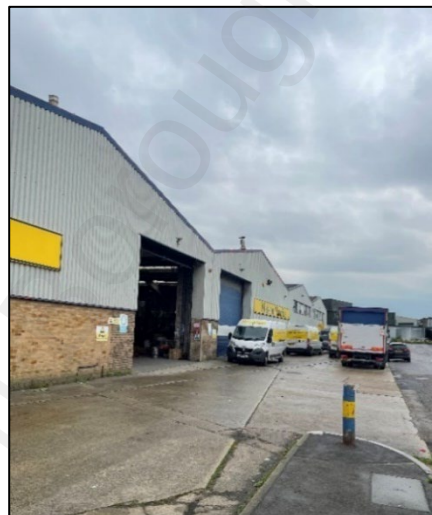
Buildings located in the north-western portion of the red line boundary
